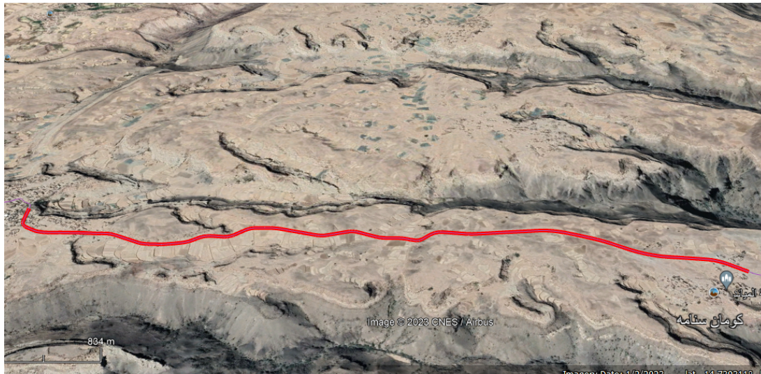
Figure 6 Road track from 5+000 km to 9+000 km
