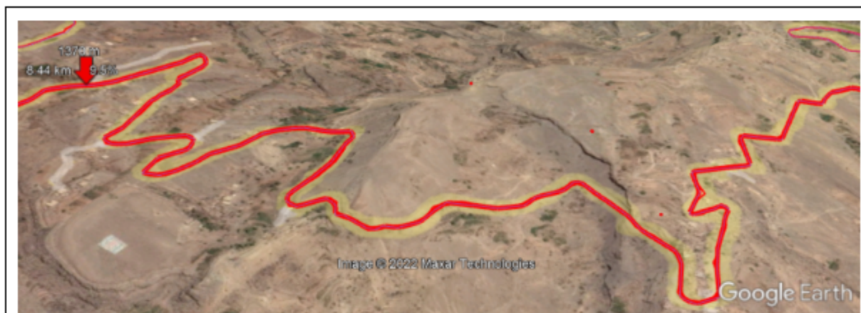
Figure 5 Road track from 4+200 km to 8+440 Km, google map.
