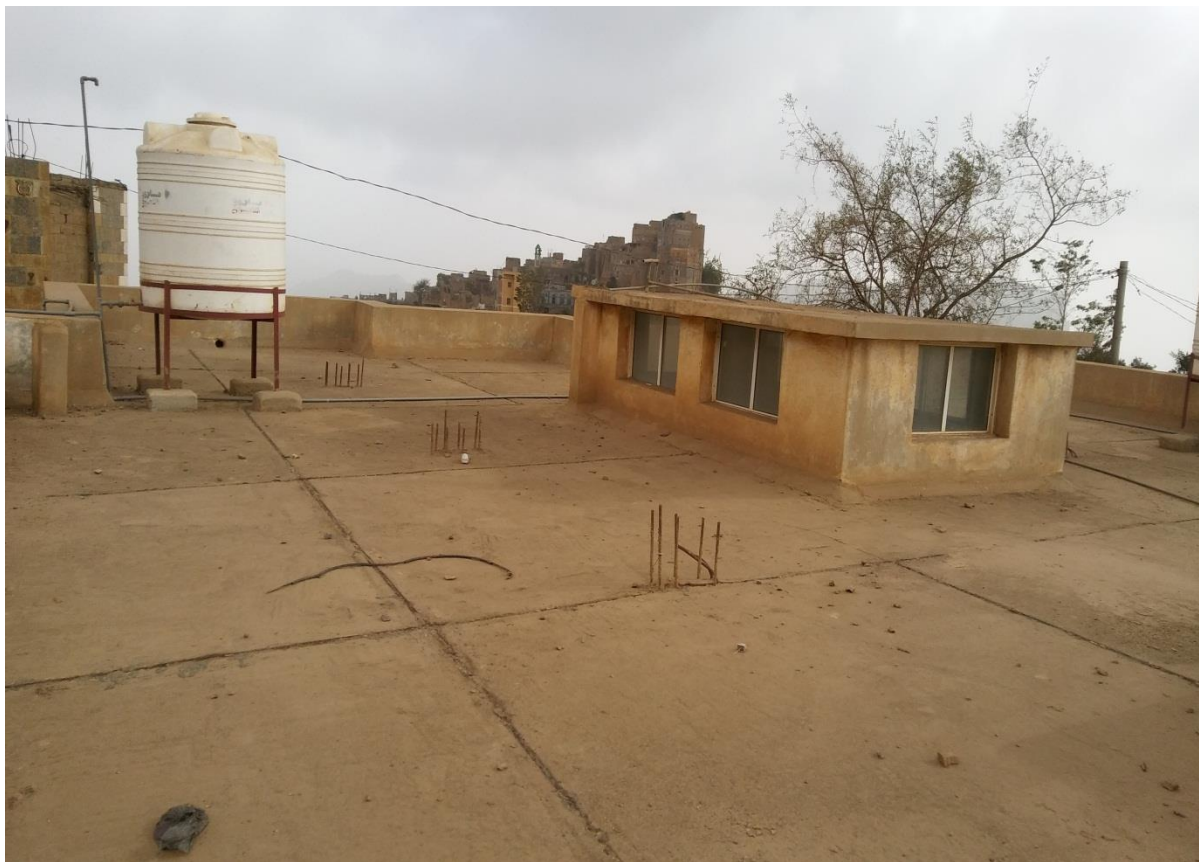
BANI MOJAI'E HEALTH CENTER Rooftop
