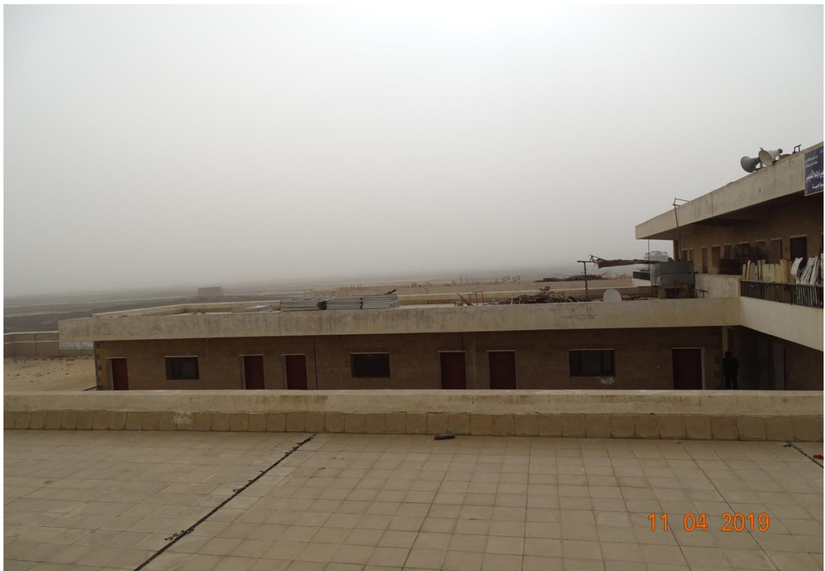
AL-SHAHEED AL-QUDAMI SCHOOL ROOFTOP
