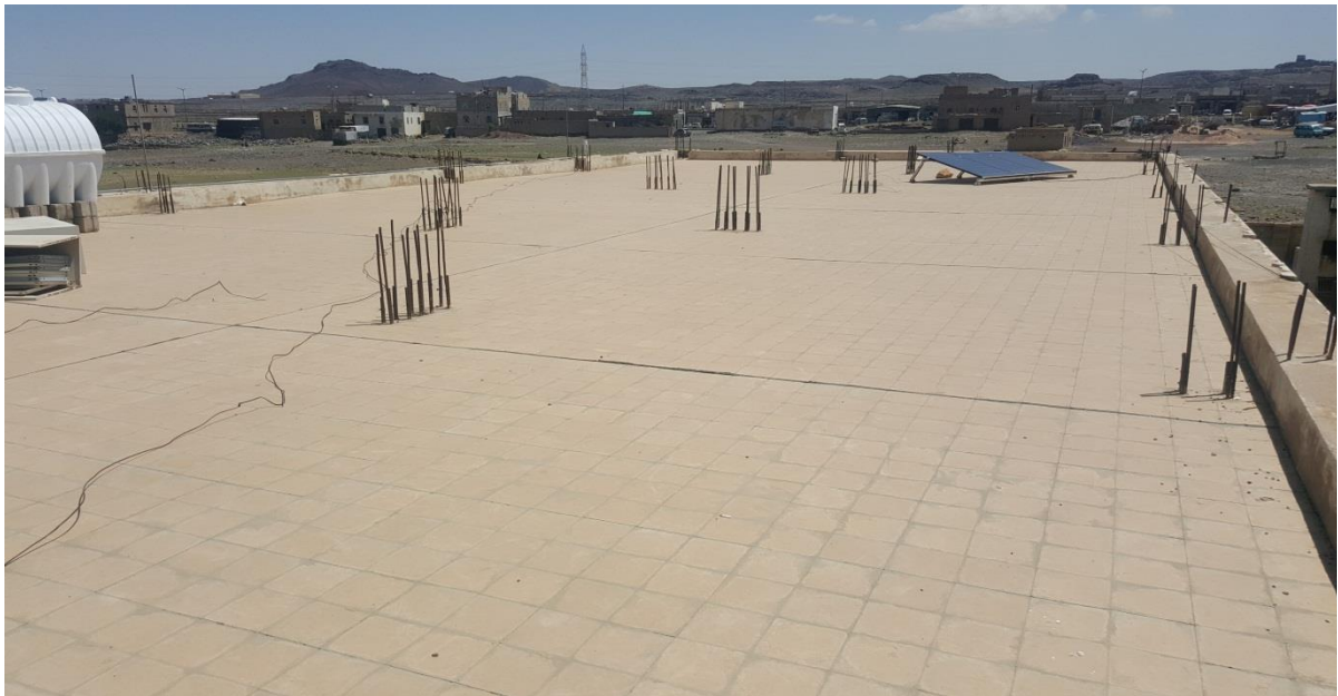
SAHAB HEALTH CENTER ROOFTOP
