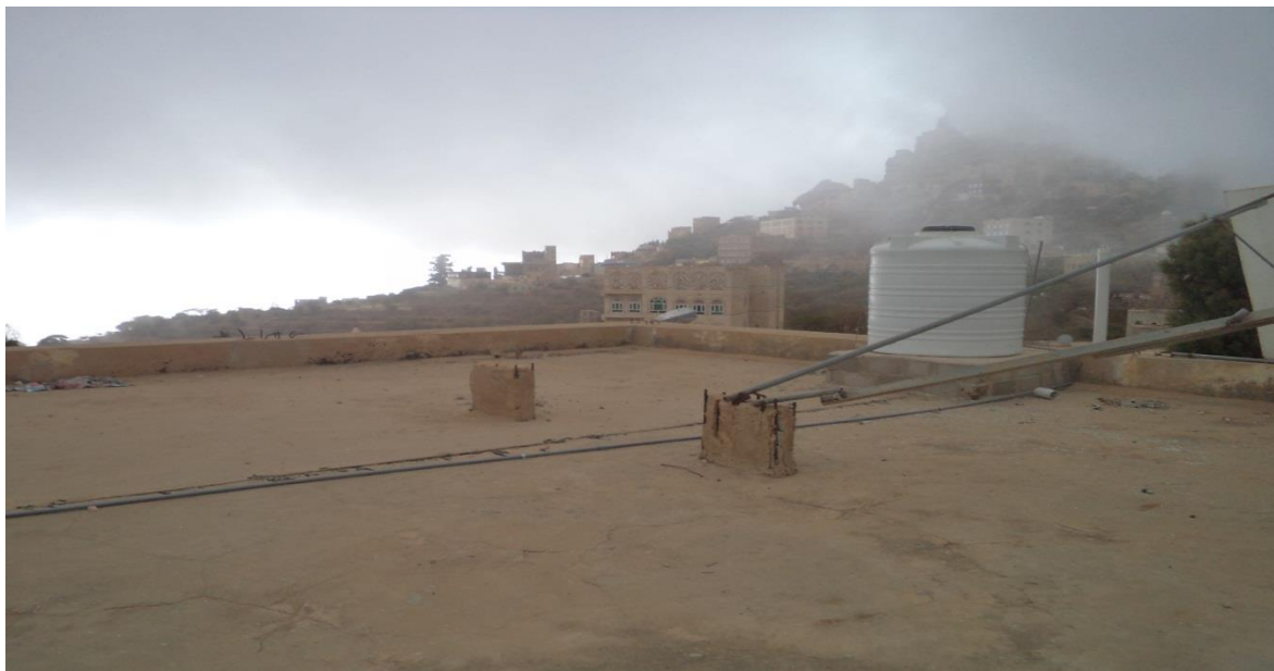
AL TAWILAH HOSPITAL ROOFTOP
