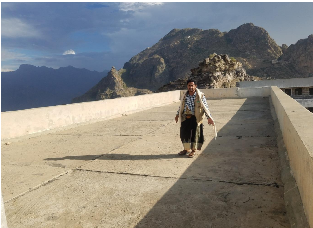
ALQUDMA EDUCATIONAL COMPLEX Rooftop
