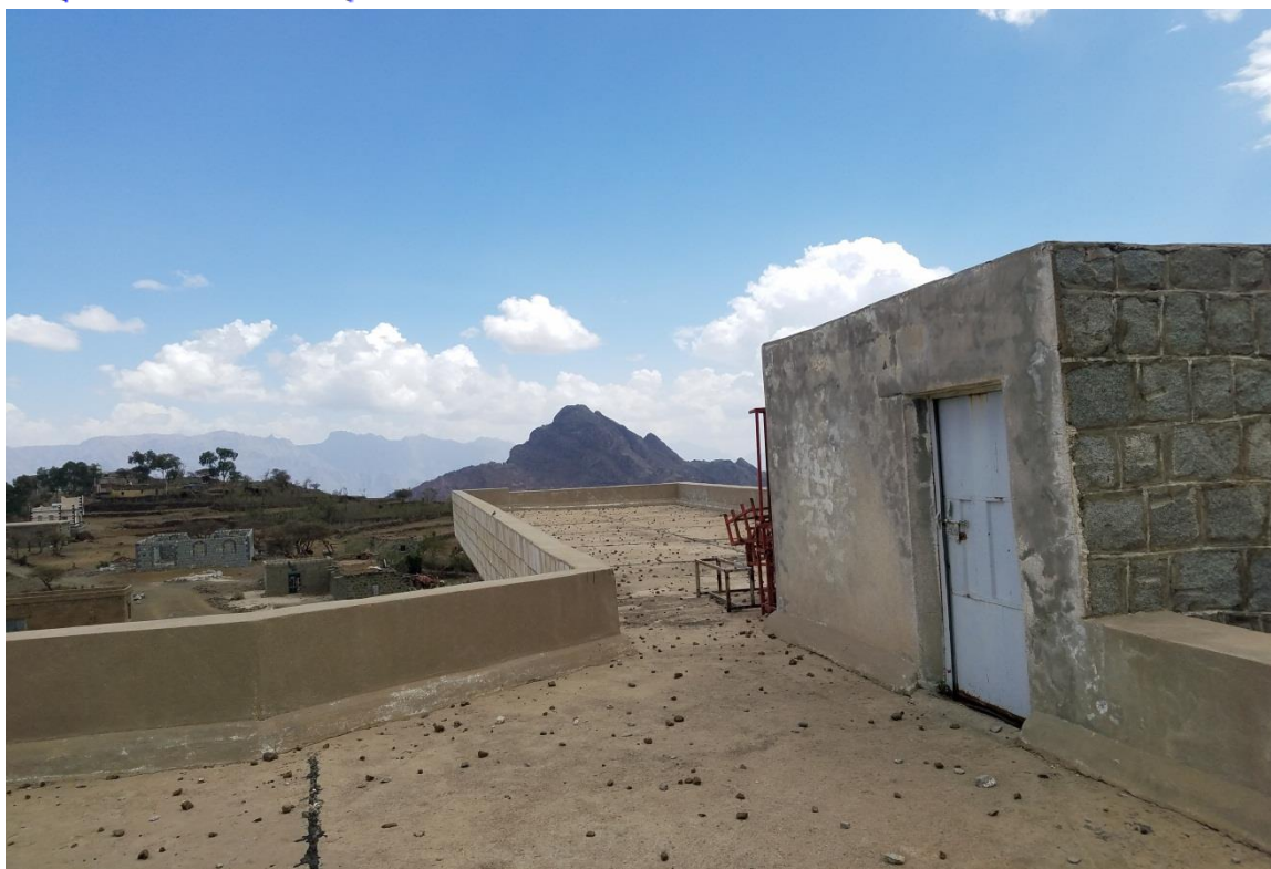
OMAR BIN ALKHATAB SCHOOL ROOFTOP
