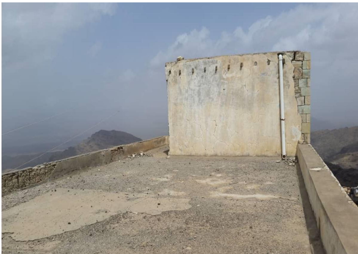
AL FALLAH SCHOOL ROOFTOP
