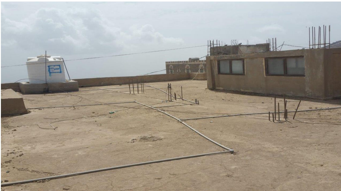
ALMASAJID HEALTH CENTER ROOFTOP
