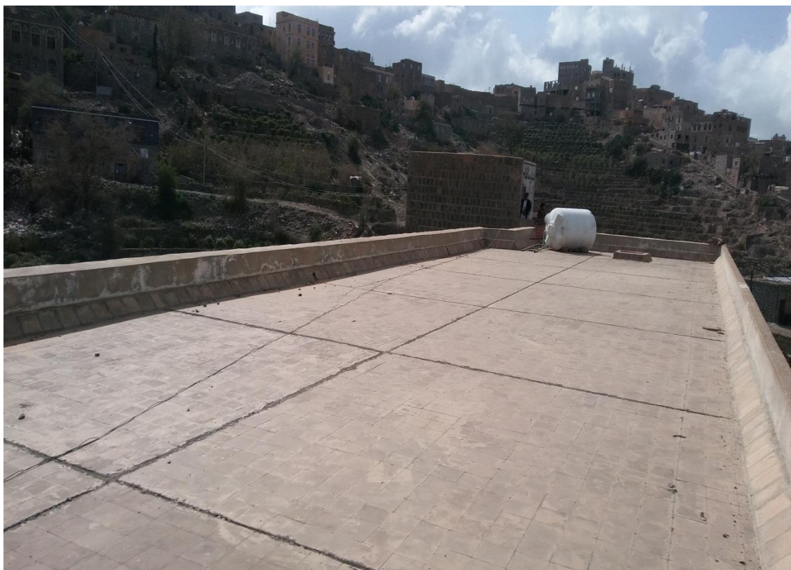
ALFLAH SCHOOL ROOFTOP
