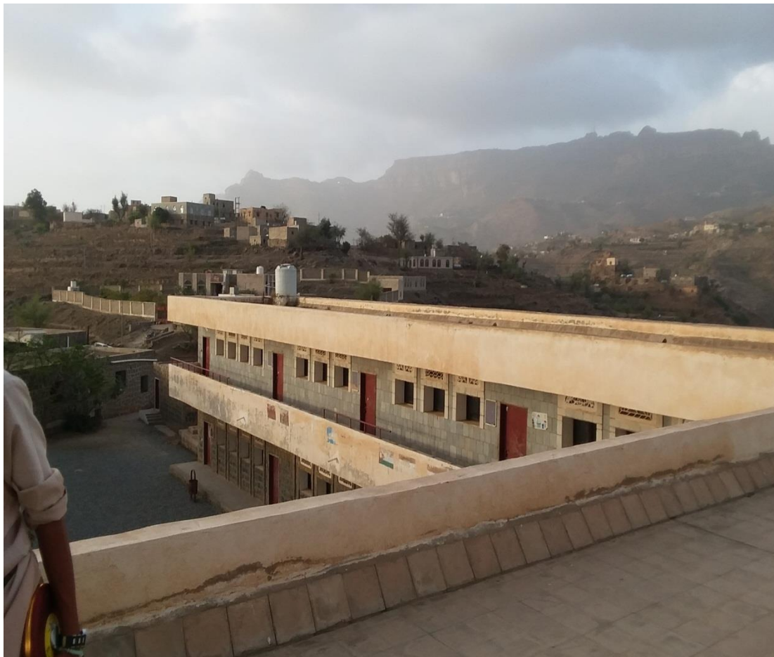
ALNASR BANI AOQAB SCHOOL ROOFTOP
