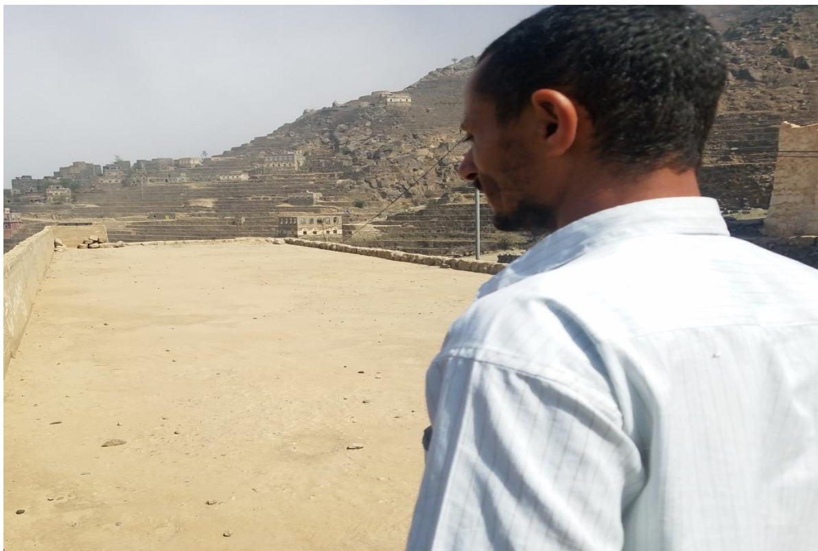
22 MAY SCHOOL Rooftop
