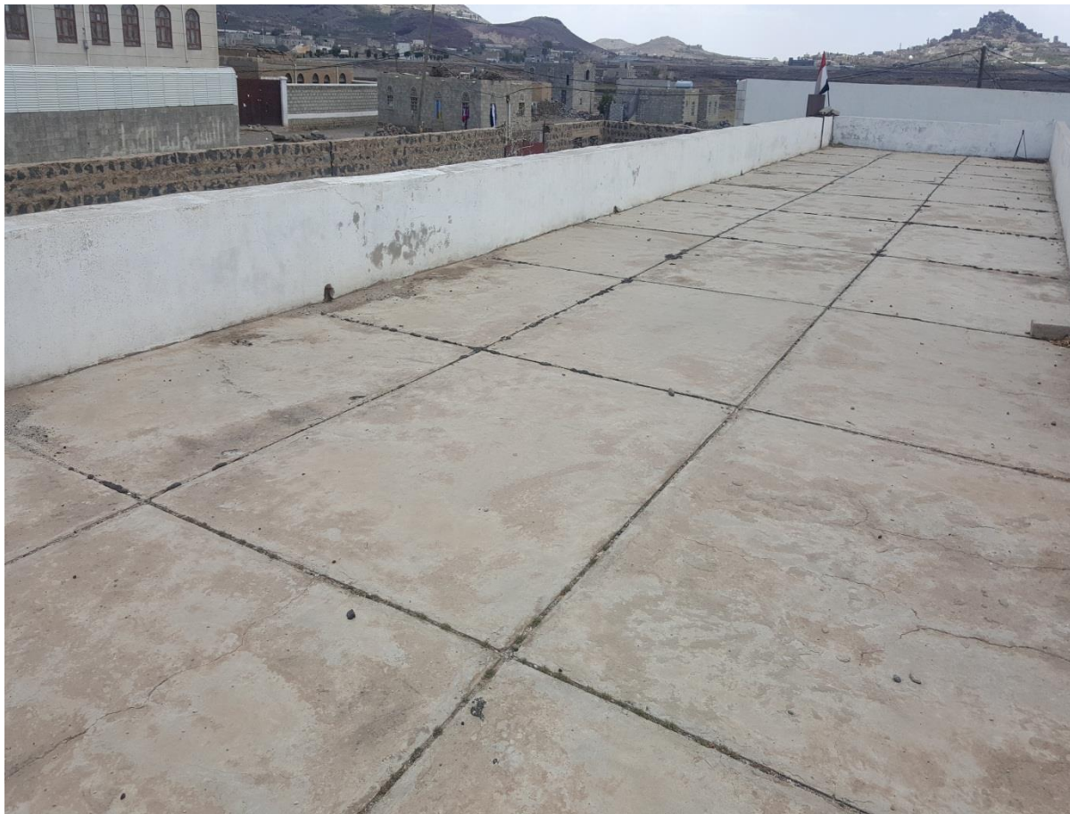
AL-RAHABI SCHOOL ROOFTOP
