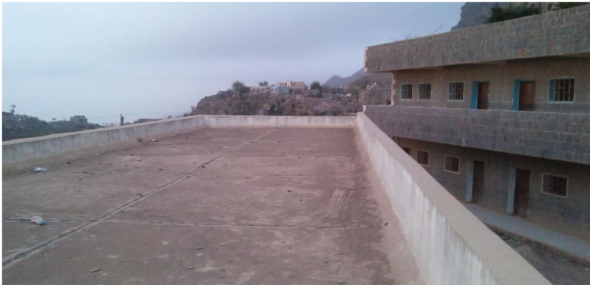
KHADIJAH SCHOOL ALMEFTAH ROOFTOP
