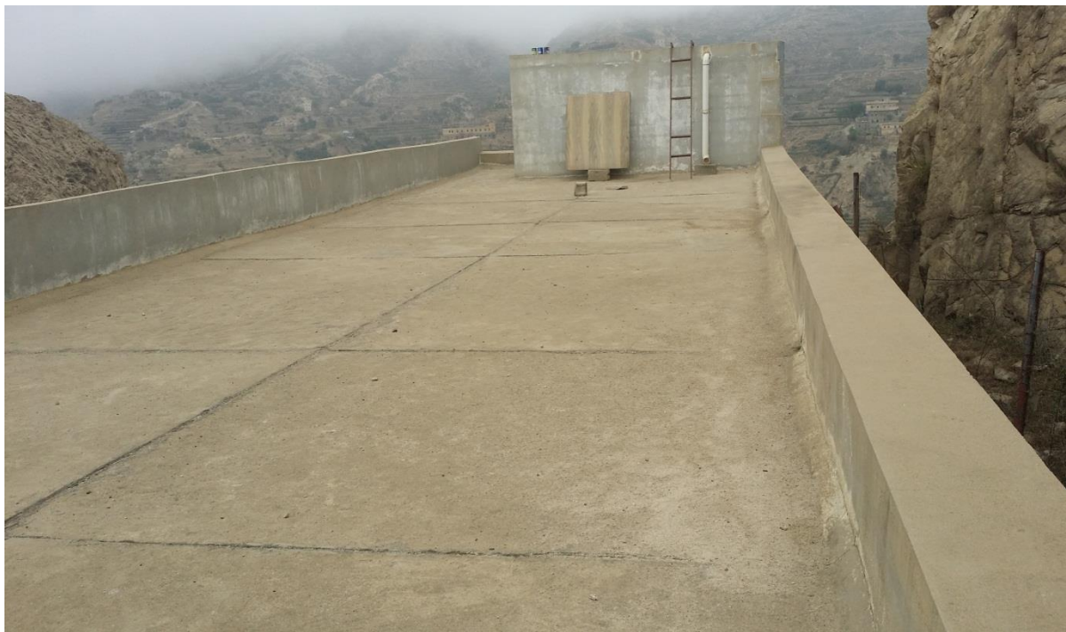
ALSALEH SCHOOL ROOFTOP
