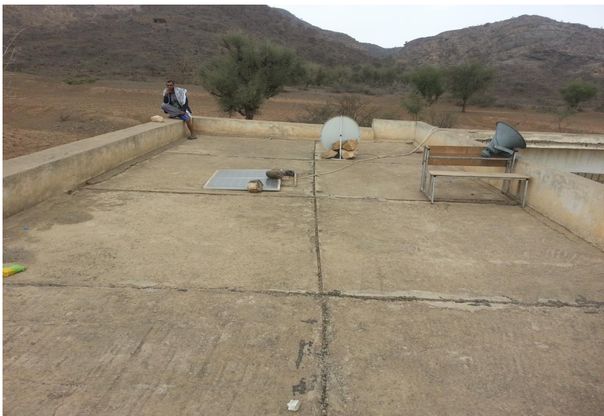
21SEPTEMBER SCHOOL ROOFTOP
