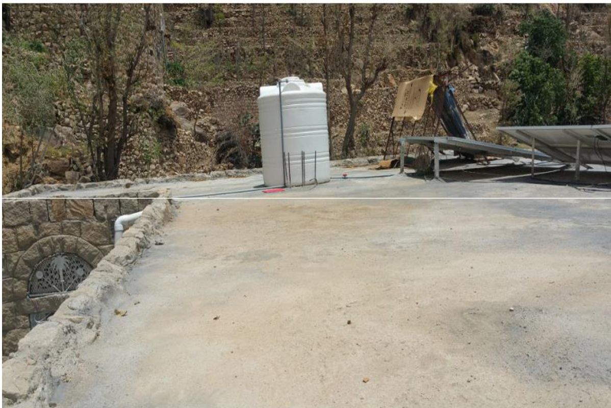
AL YARMOOK HEALTH CENTER ROOFTOP
