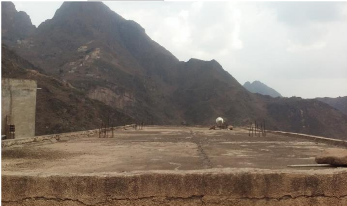
ALNASER SCHOOL ROOFTOP
