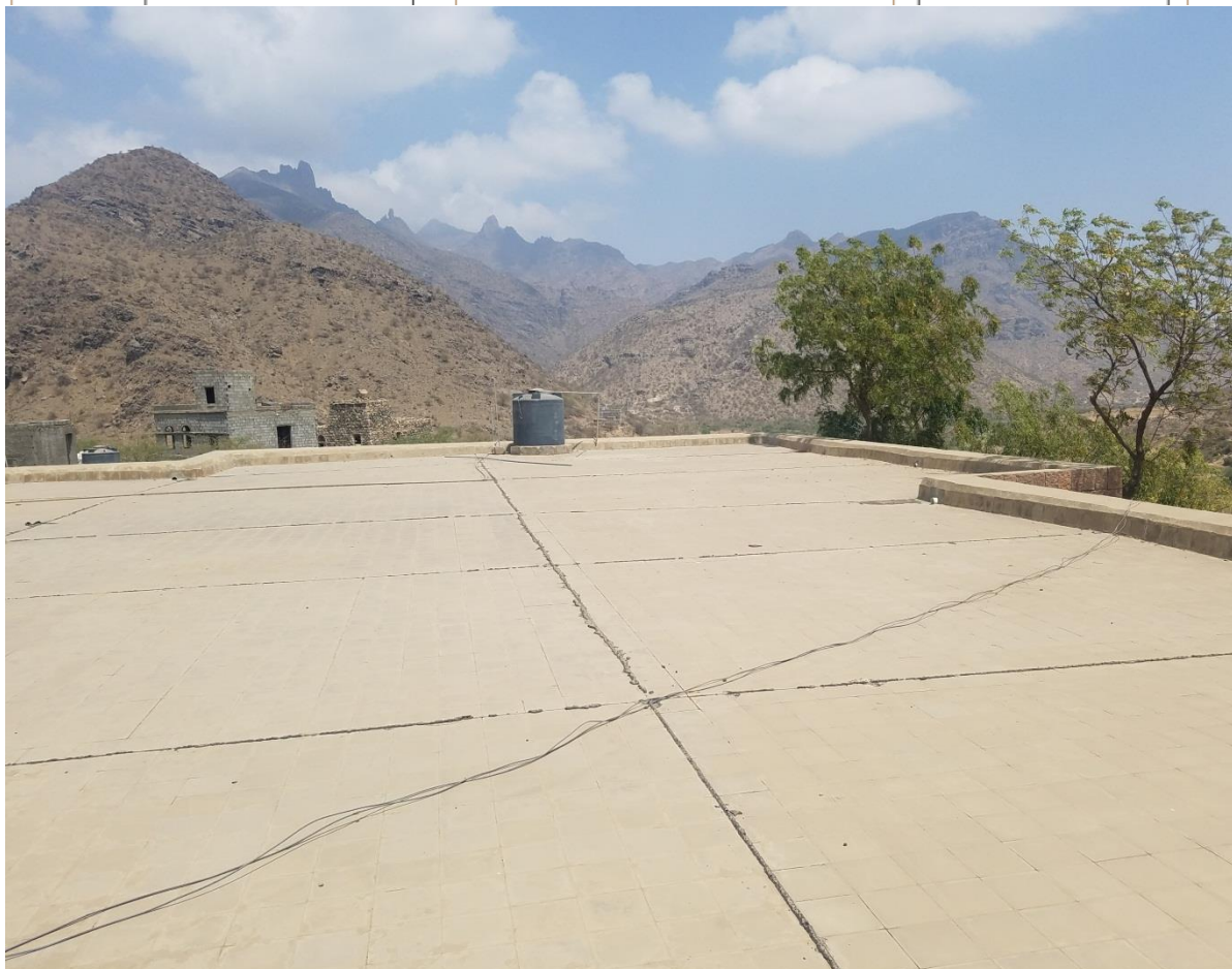
ALMETHAQ RURAL HOSPITAL ROOFTOP
