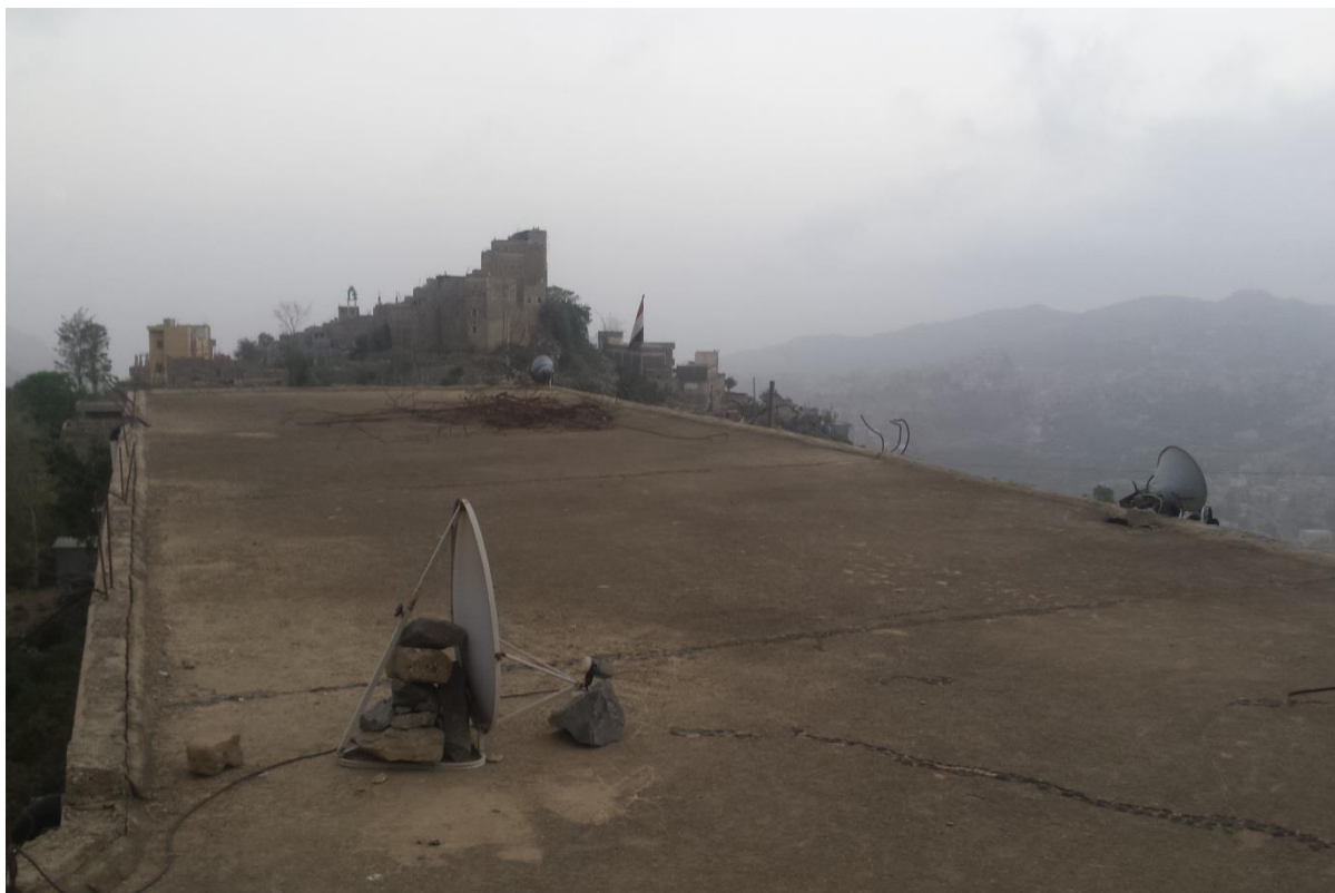
AL HASSANAIN SCHOOL ROOFTOP
