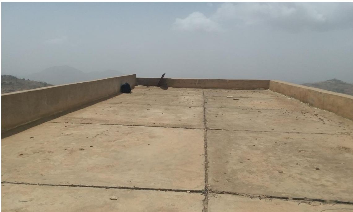
GHANEM SCHOOL Rooftop
