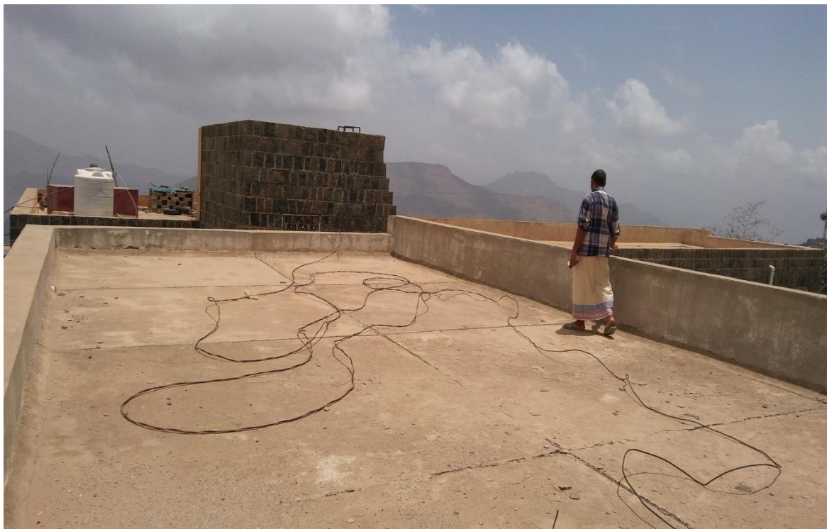
AL ZAHRA'A SCHOOL ROOFTOP
