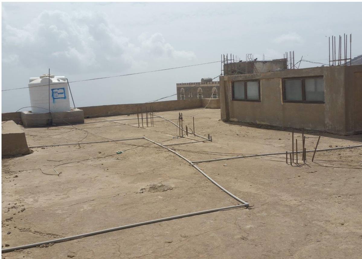
BANI SHAMAKH HEALTH CENTER Rooftop
