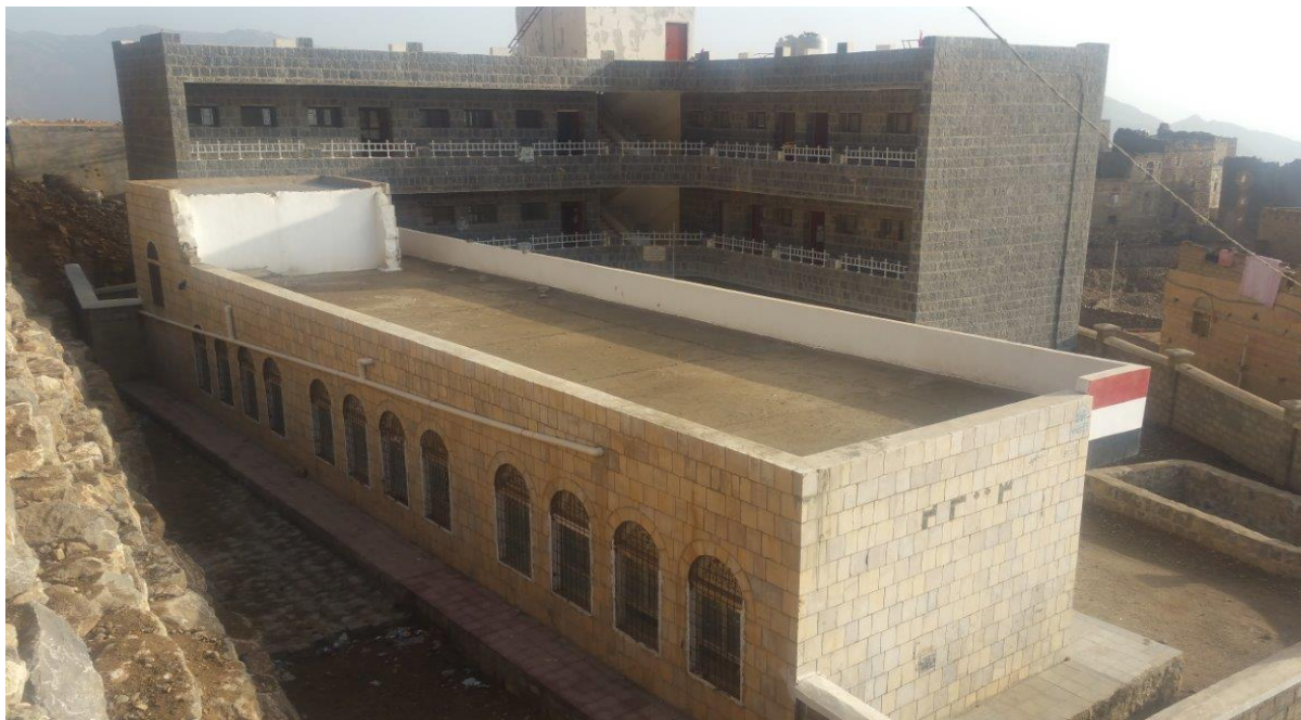
ALWAHDAH SCHOOL ROOFTOP
