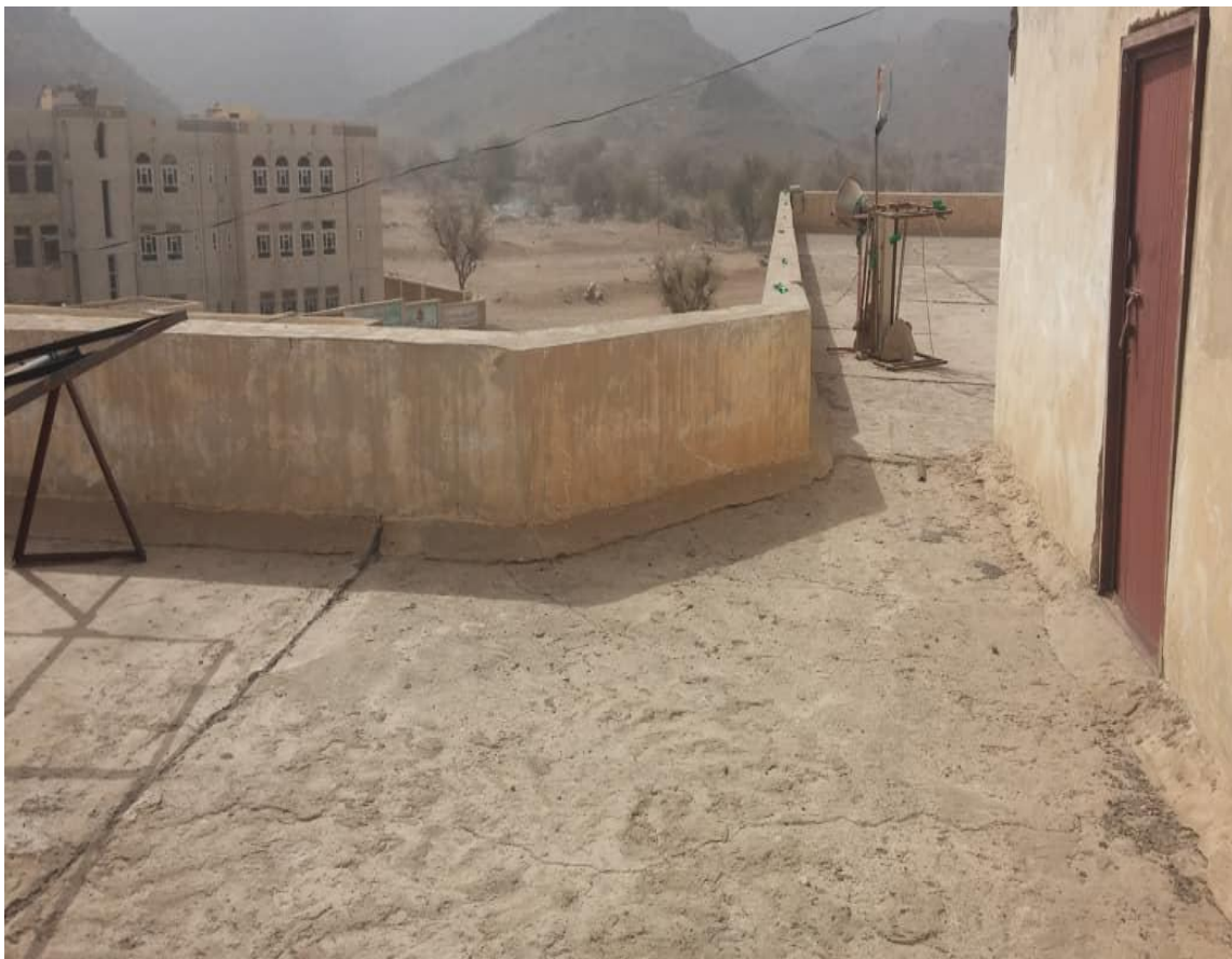
ALNOOR SCHOOL ROOFTOP
