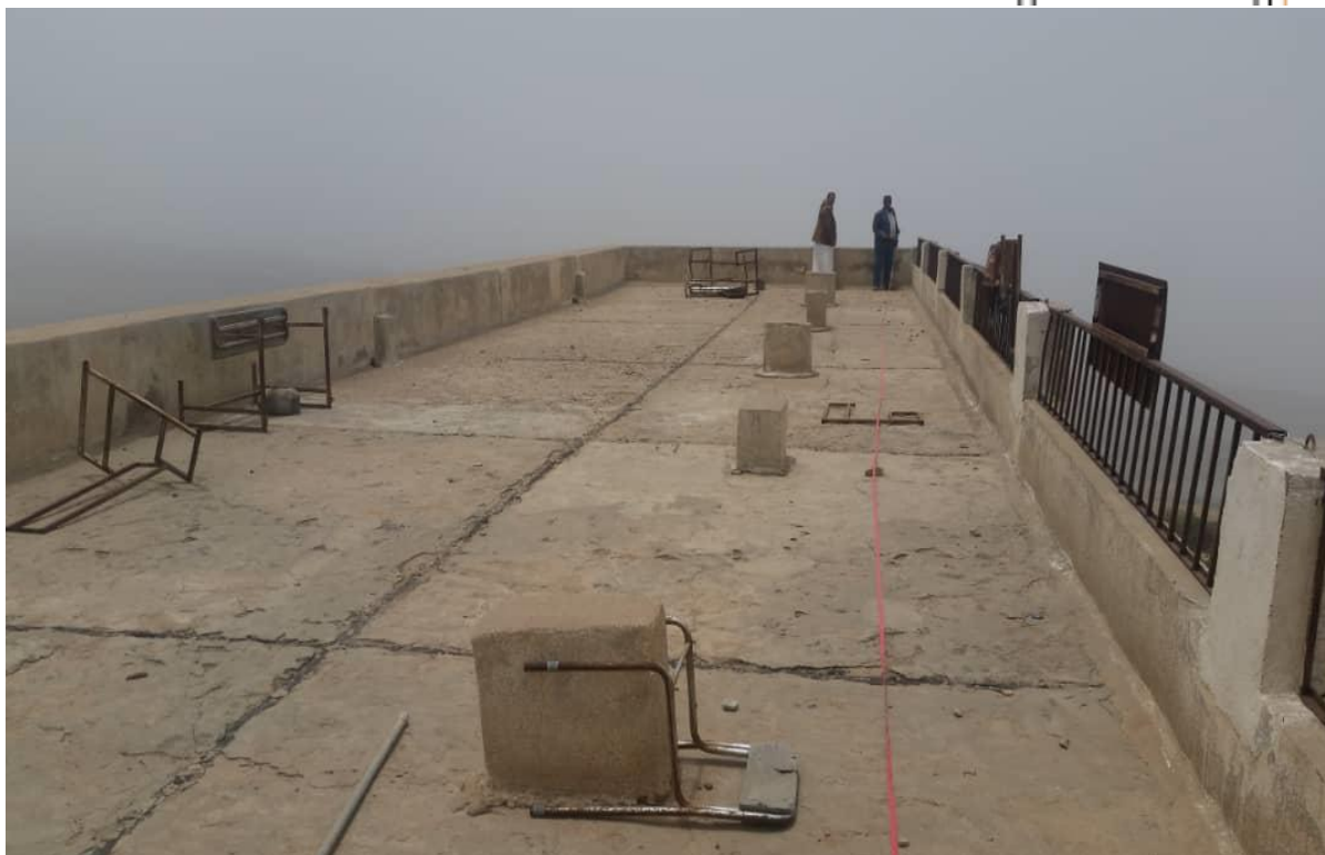
HAROON AL-RASHEED SCHOOL ROOFTOP
