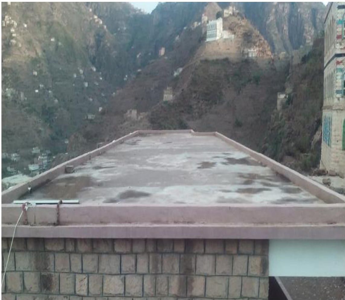
ALFATEH SCHOOL - ALJAFARIAH ROOFTOP
