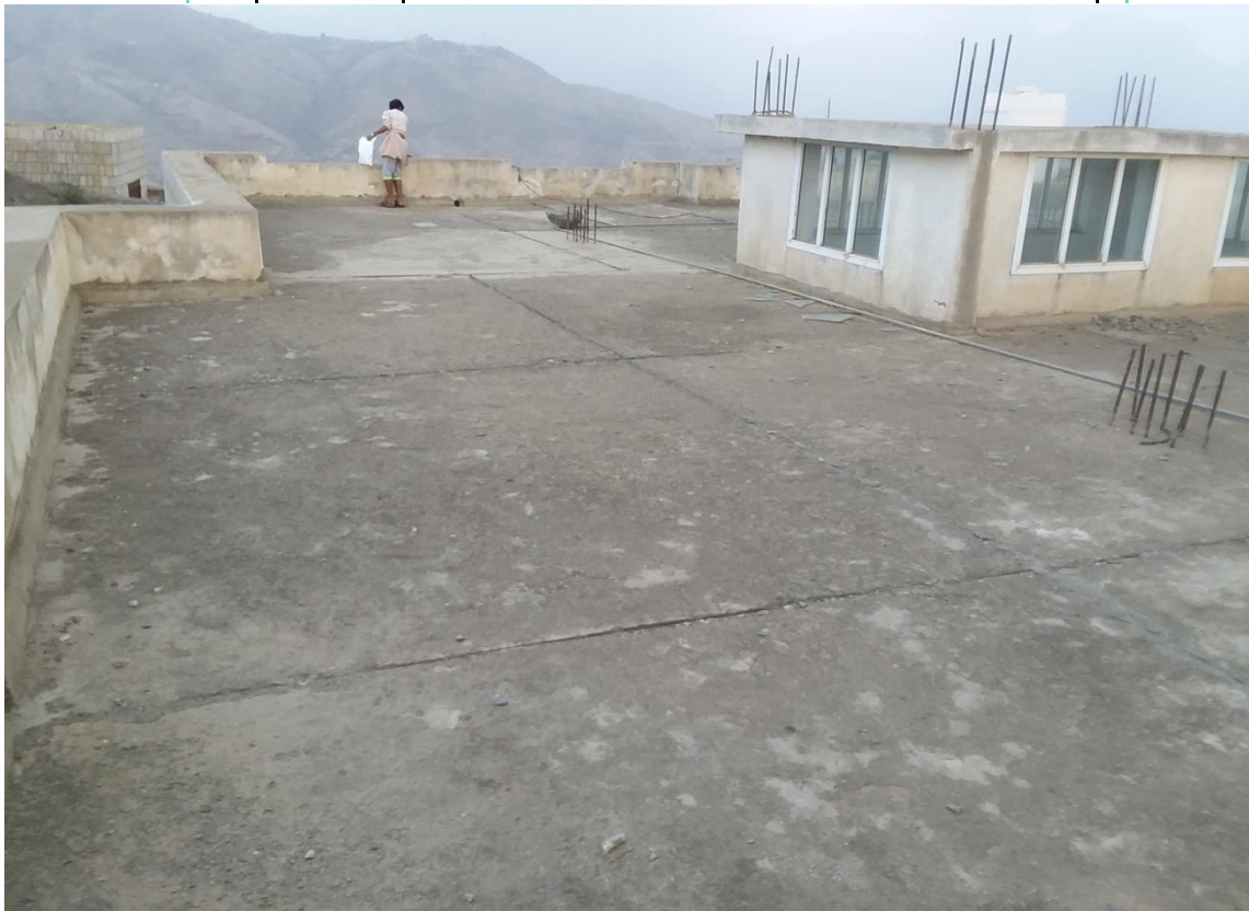
BANI OQAB HEALTH CENTER ROOFTOP
