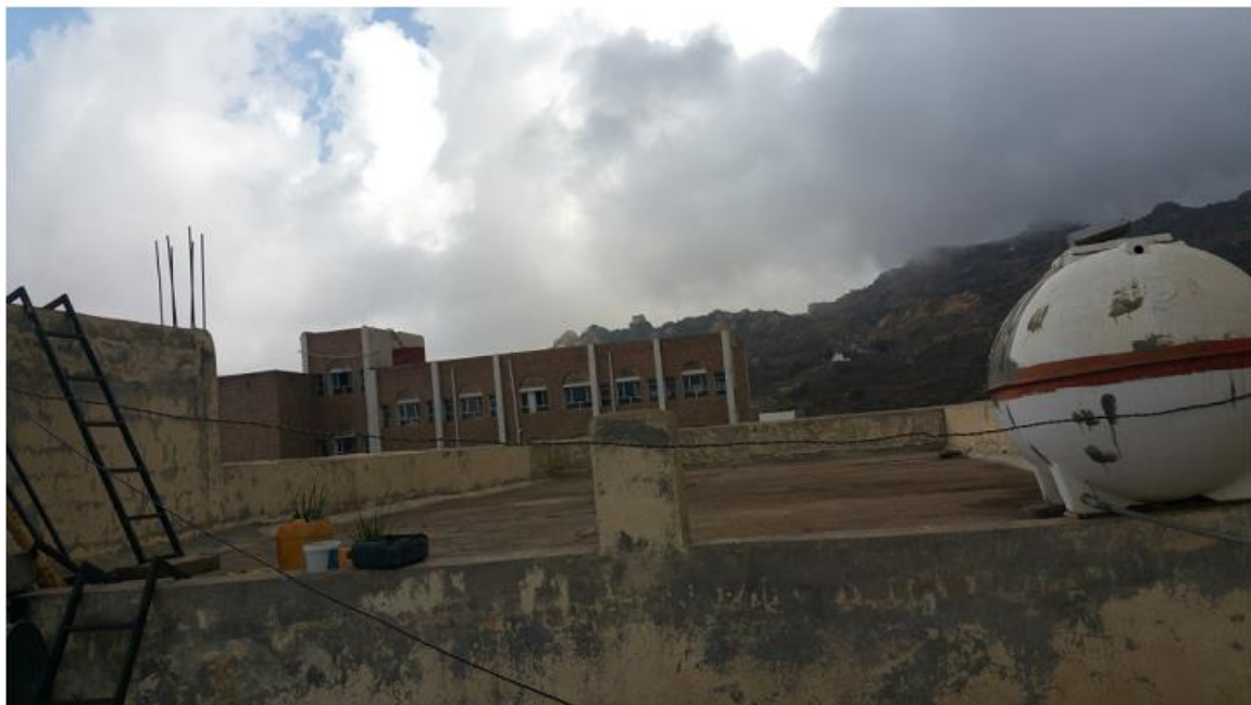
ALFATEH SCHOOL - ALGABEEN ROOFTOP
