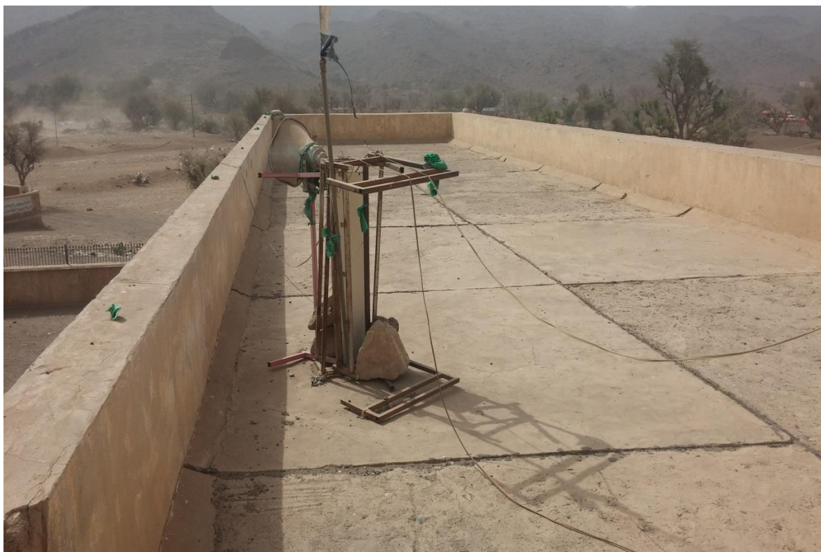
AL-NOUR SCHOOL ROOFTOP
