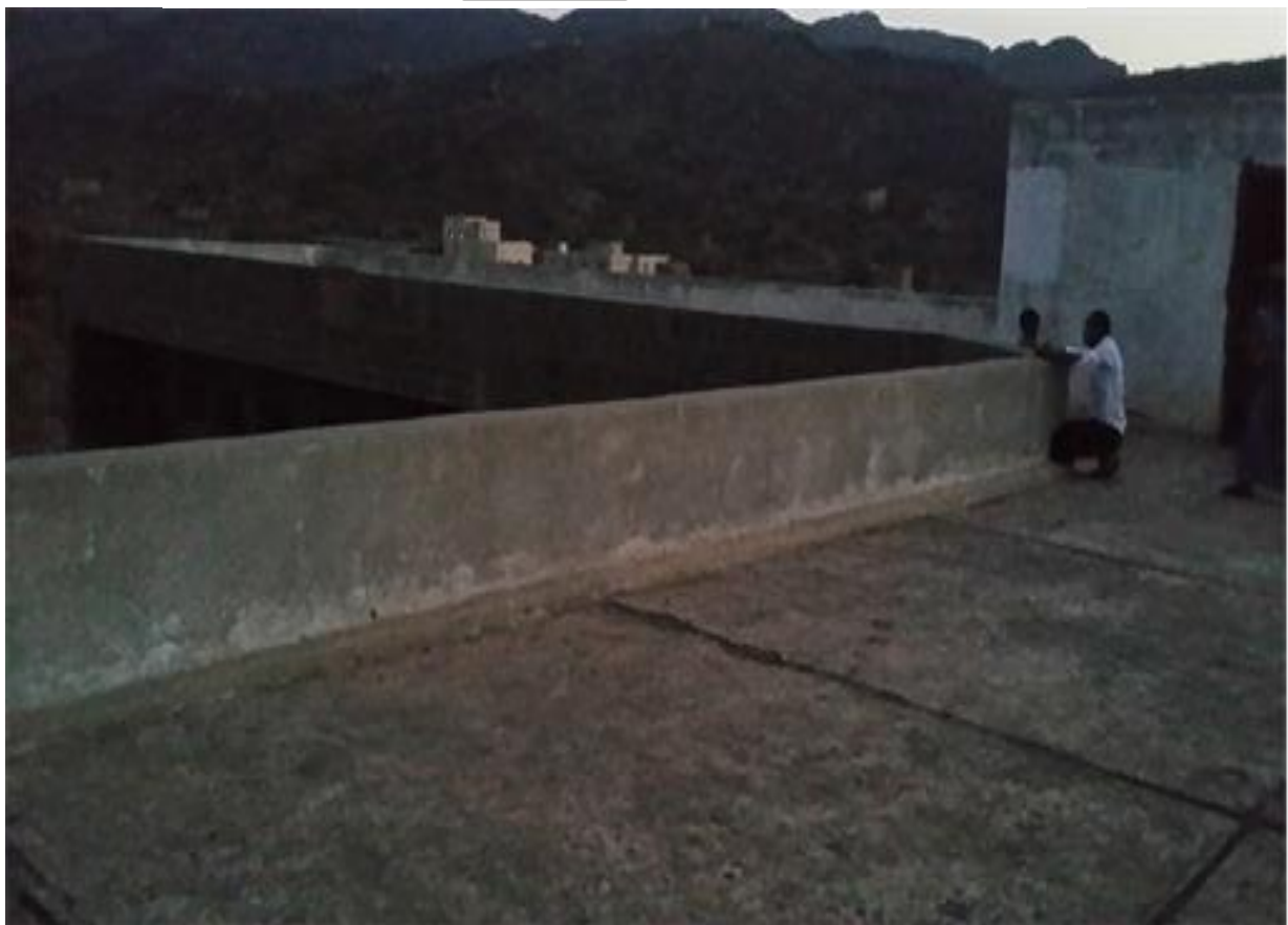
ALKHATWAH SCHOOL ROOFTOP
