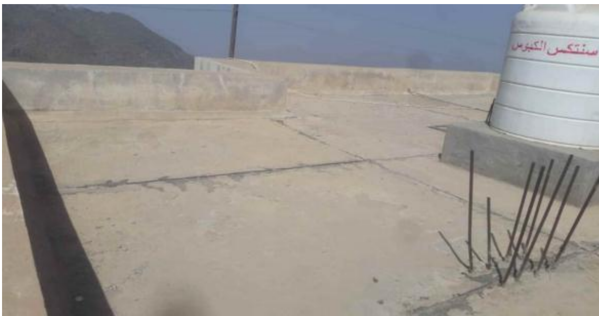
Bait Al Modai Health Center Rooftop
