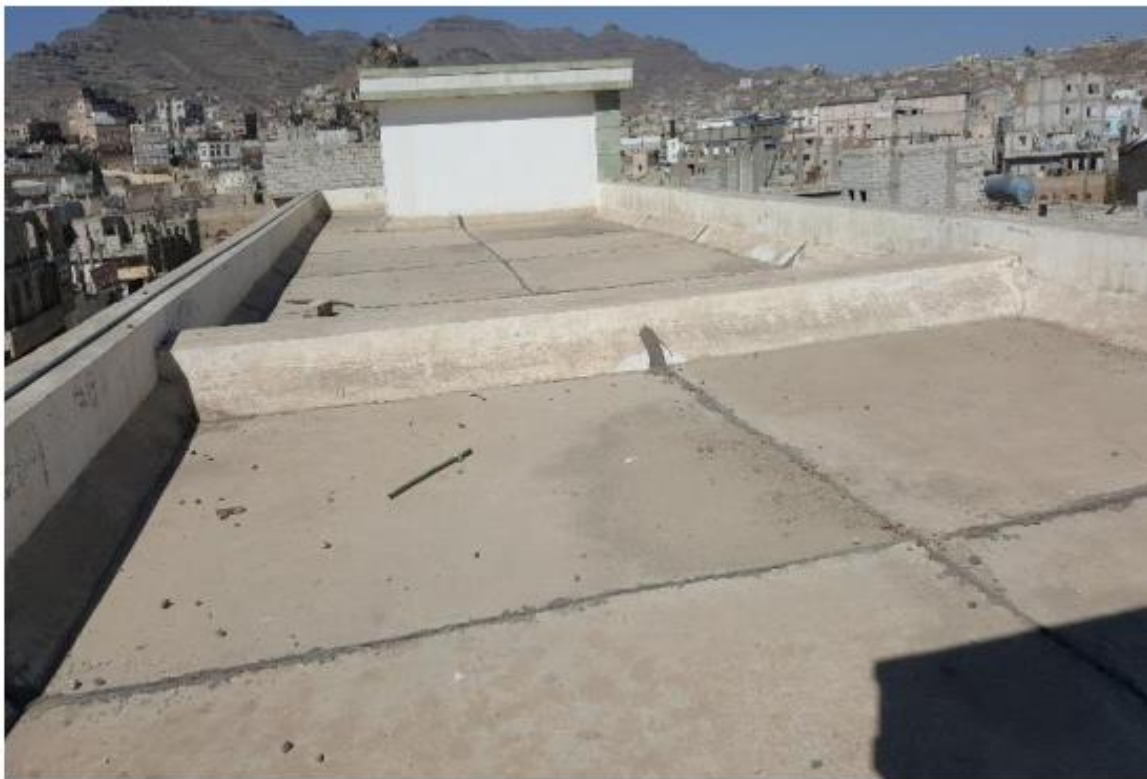
KHADIGAH SCHOOL Rooftop
