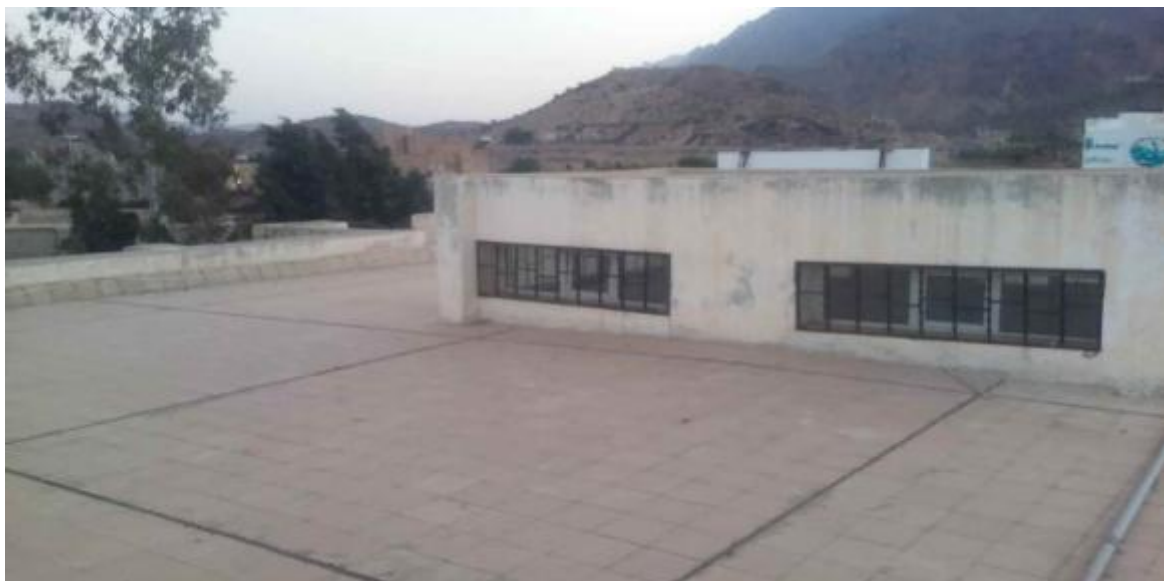
AL-Sabet Health Center Rooftop
