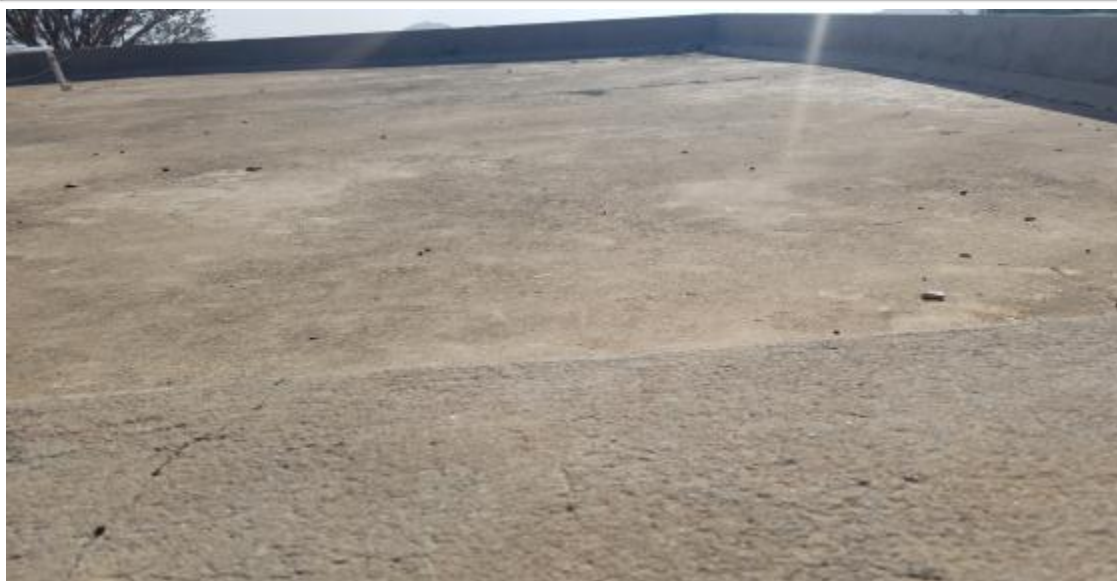
THEBA HEALTH CENTER Rooftop
