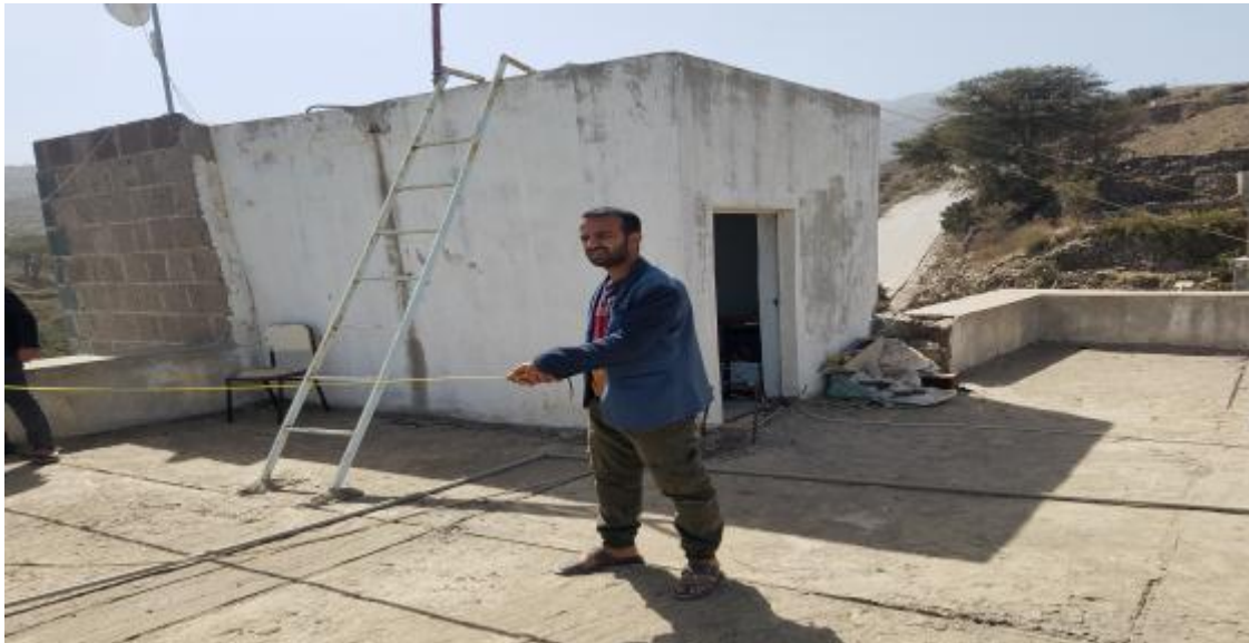
SOUQ ALRABOOA HEALTH CENTER Rooftop
