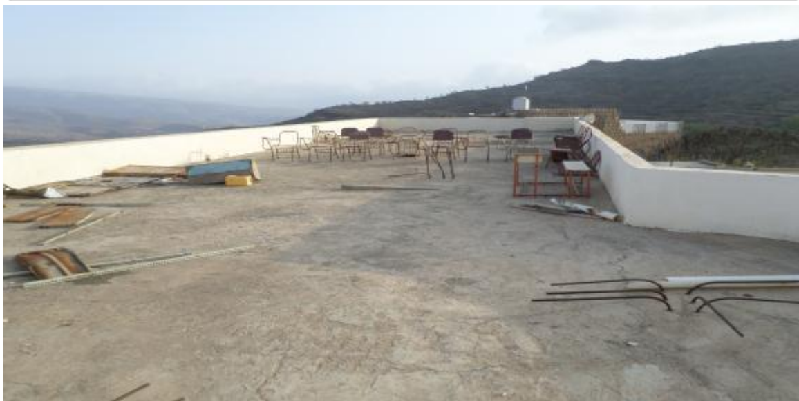
AL-WAHDA SCHOOL Rooftop
