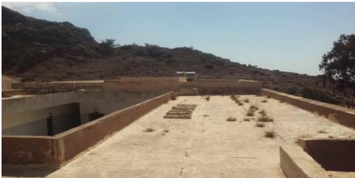
AT-TURBAH SCHOOL ROOFTOP
