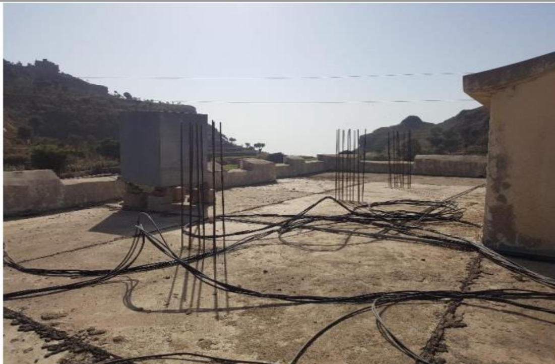
HADHAR HEALTH CENTER Rooftop
