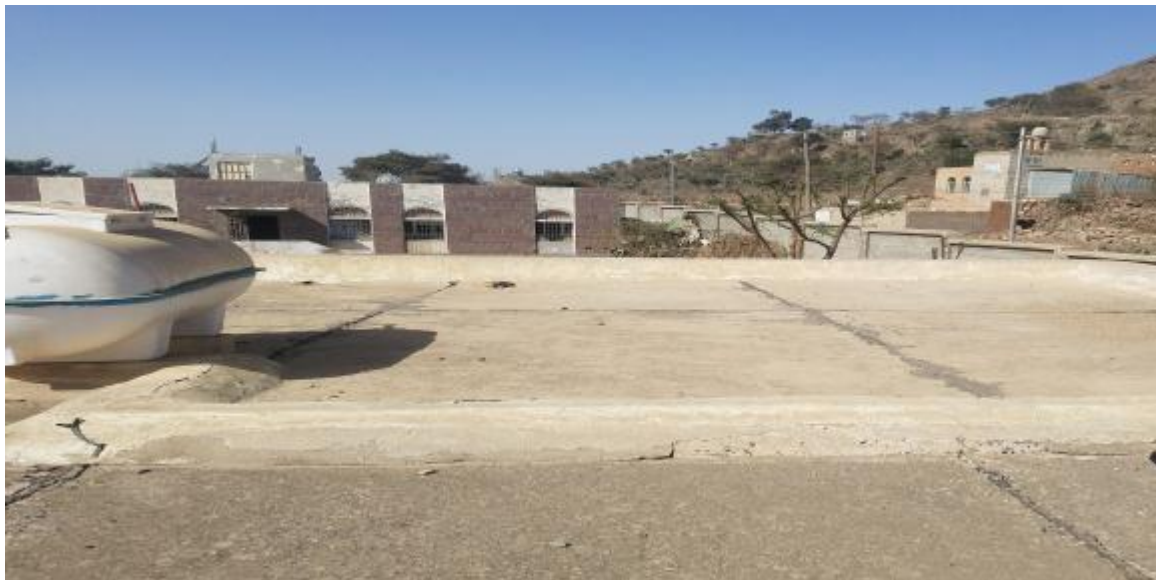
DALMA HUBAISH HEALTH CENTER Rooftop
