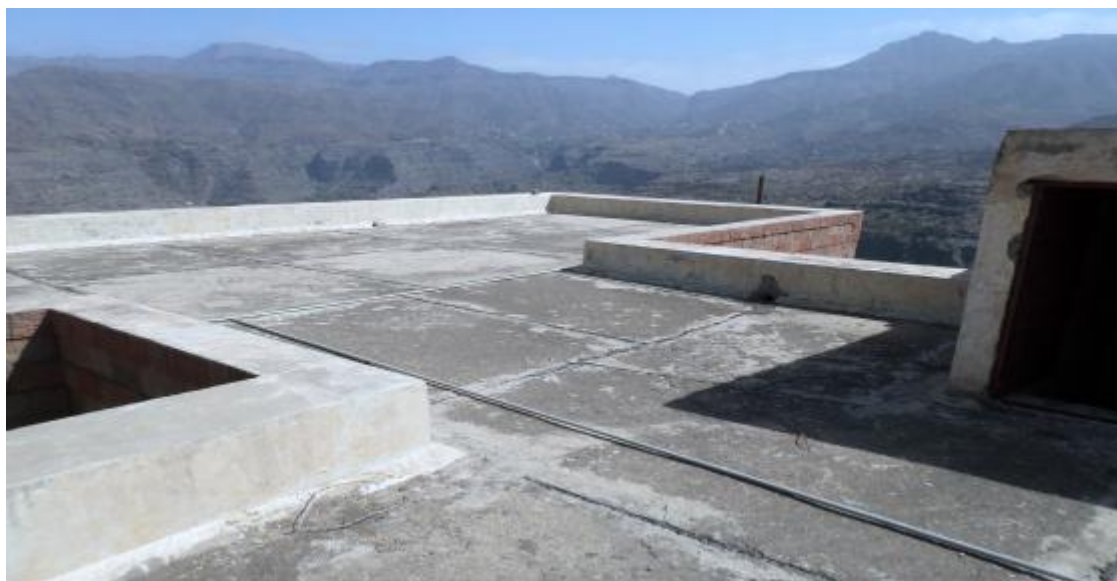
AL-OSAILA_A HEALTH CENTER Rooftop
