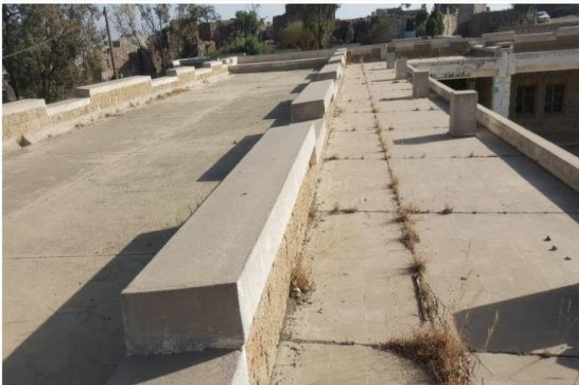
AL SHAHEED ALERIANI SCHOOL Rooftop
