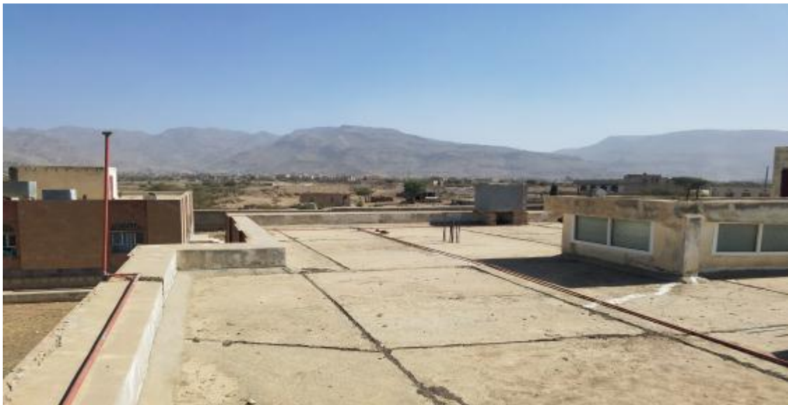
AL SAIH HEALTH CENTER Rooftop
