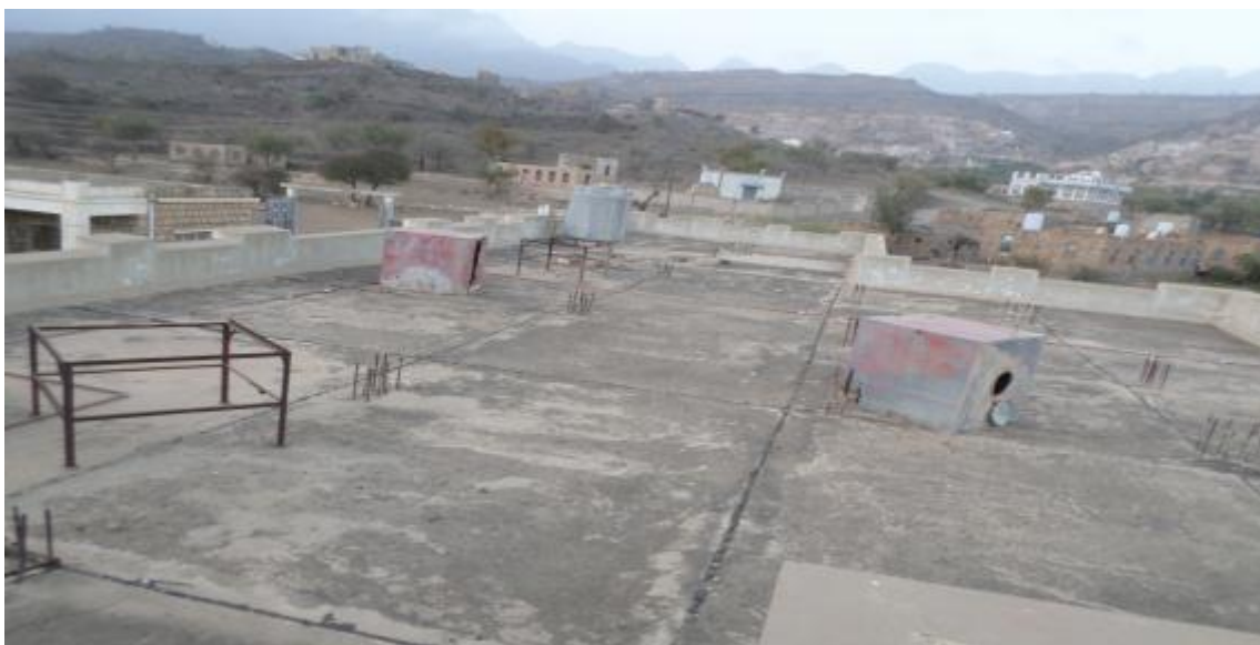
ALSHAHEED ALI SALEH BANI SHAIBAH HEALTH CENTER Rooftop
