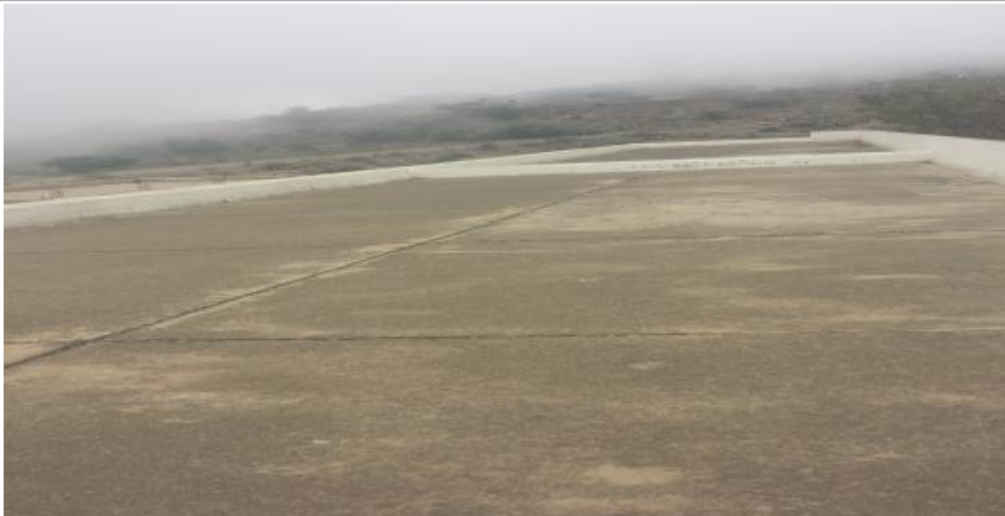
ALERSHAD SCHOOL Rooftop
