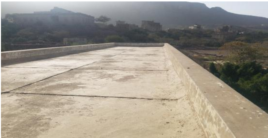
AL ESHRAK SCHOOL Rooftop
