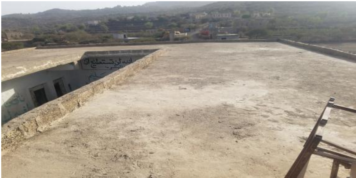
AL LUQIAH SCHOOL Rooftop
