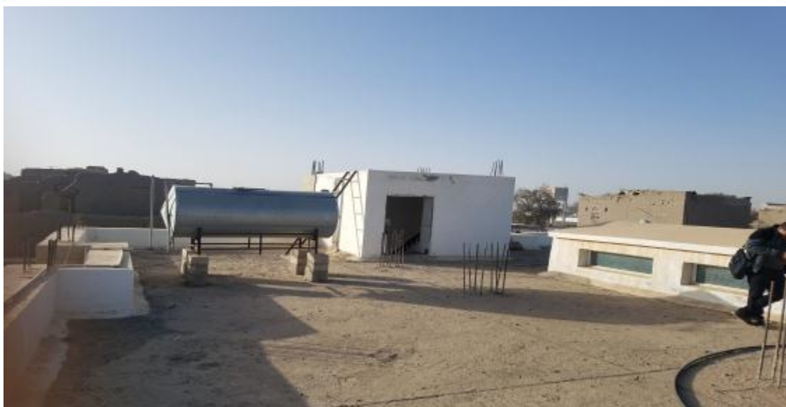
AL KHAREBAH HEALTH CENTER Rooftop
