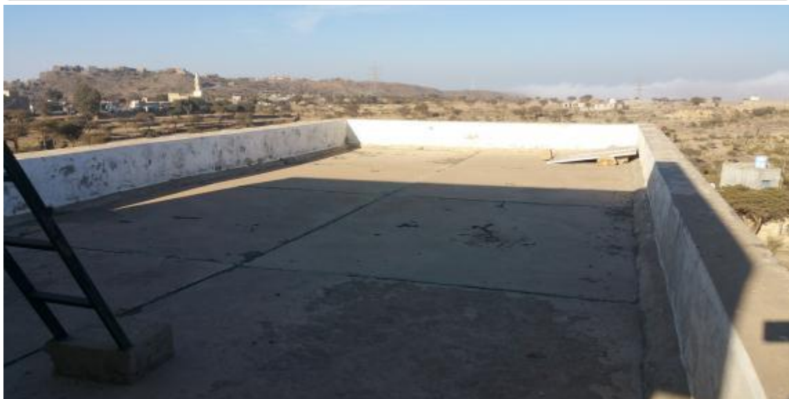
JEEL AL-JADEED SCHOOL Rooftop
