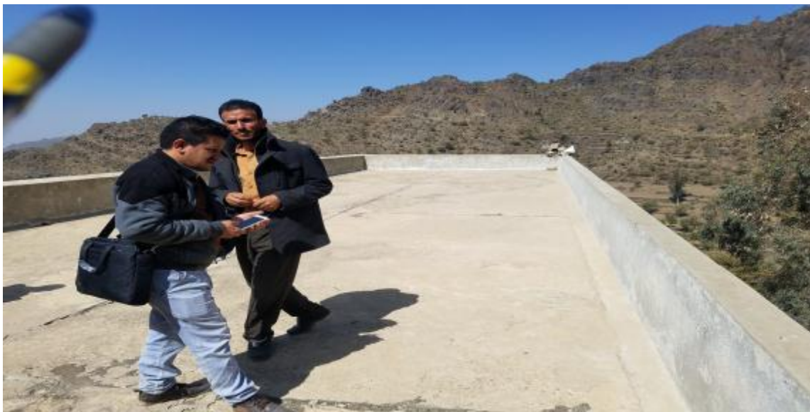
AL HASIB SCHOOL Rooftop
