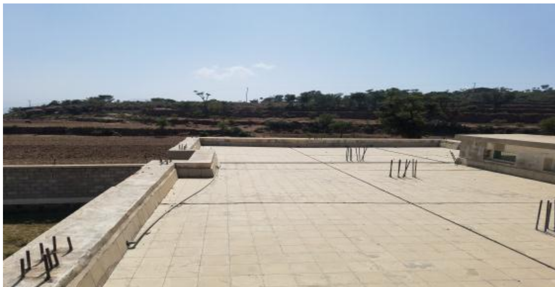
BANI SALAMAH HEALTH CENTER Rooftop
