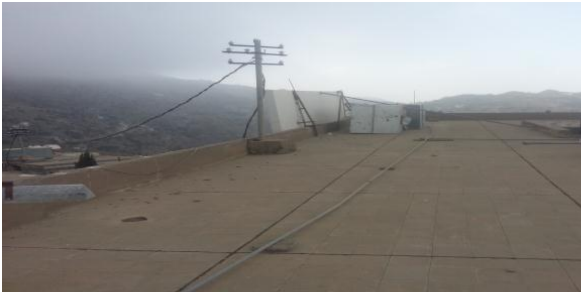
ALHATWAH HEALTH CENTER Rooftop
