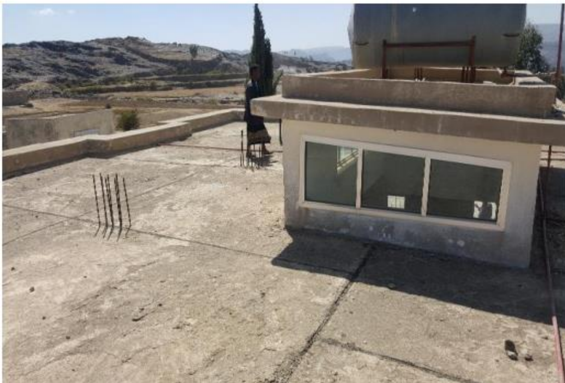
BAIT HAJINAH HEALTH CENTER Rooftop
