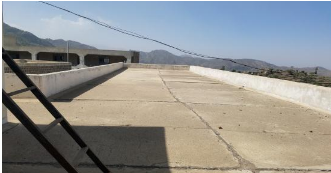
AL QADESIAH SCHOOL Rooftop
