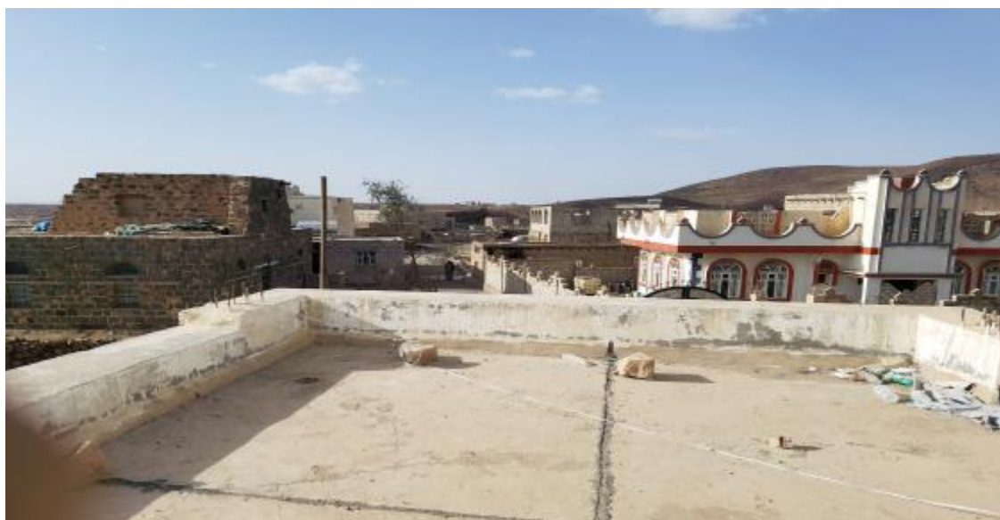
JARF ASBEEL HEALTH CENTER Rooftop
