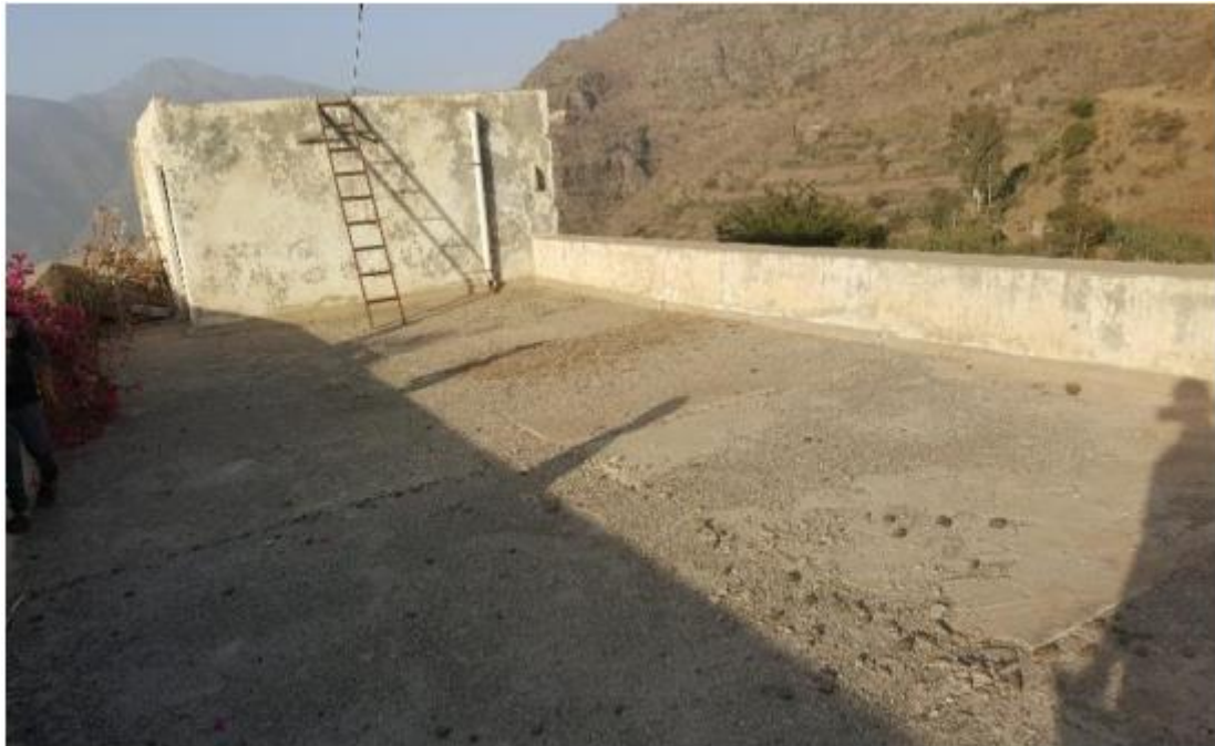
AL SHAHID SHJAA ALDEEN SCHOOL Rooftop
