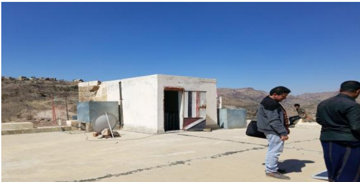
THEE ATA HEALTH CENTER Rooftop
