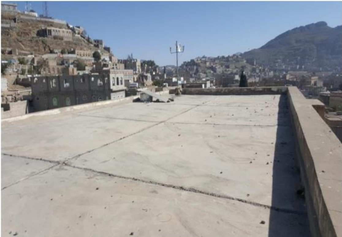
AL KHANSA SCHOOL Rooftop
