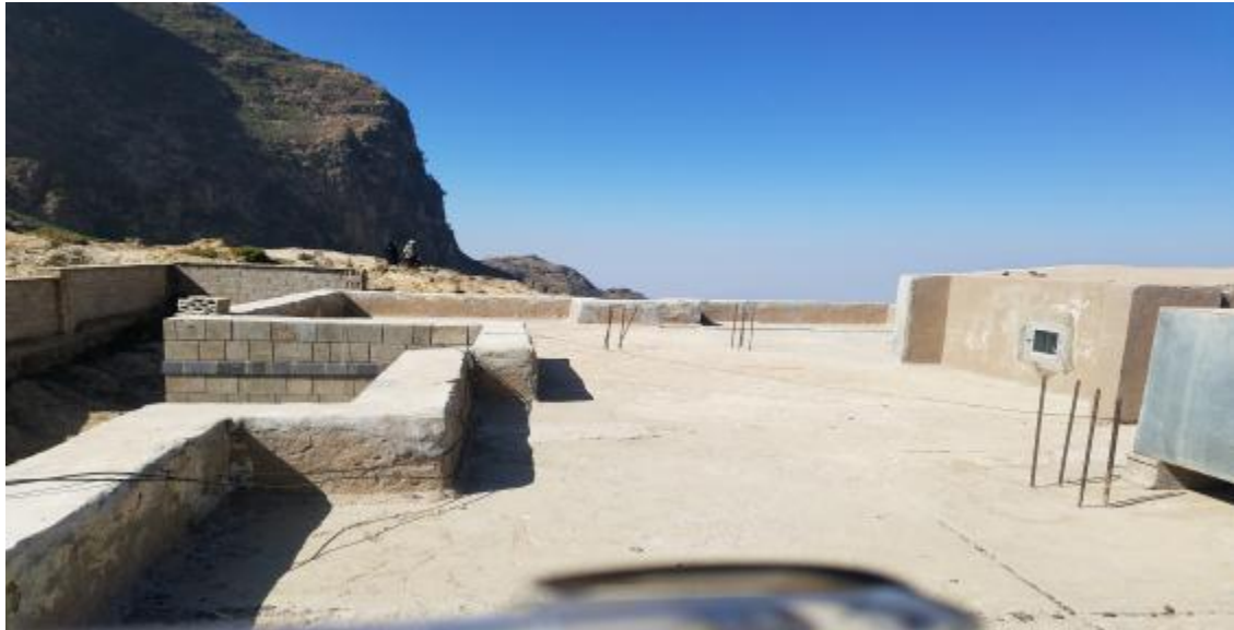
AL MAIDAN HEALTH CENTER Rooftop
