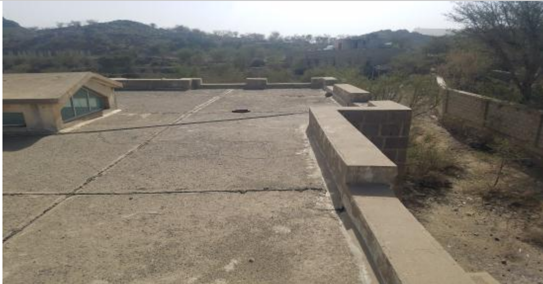
AL NAHEIAH HEALTH CENTER Rooftop
