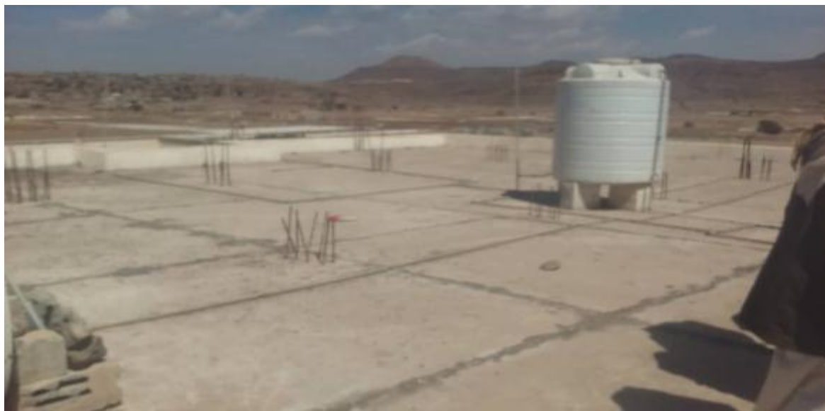
MASAOOD HEALTH CENTER Rooftop
