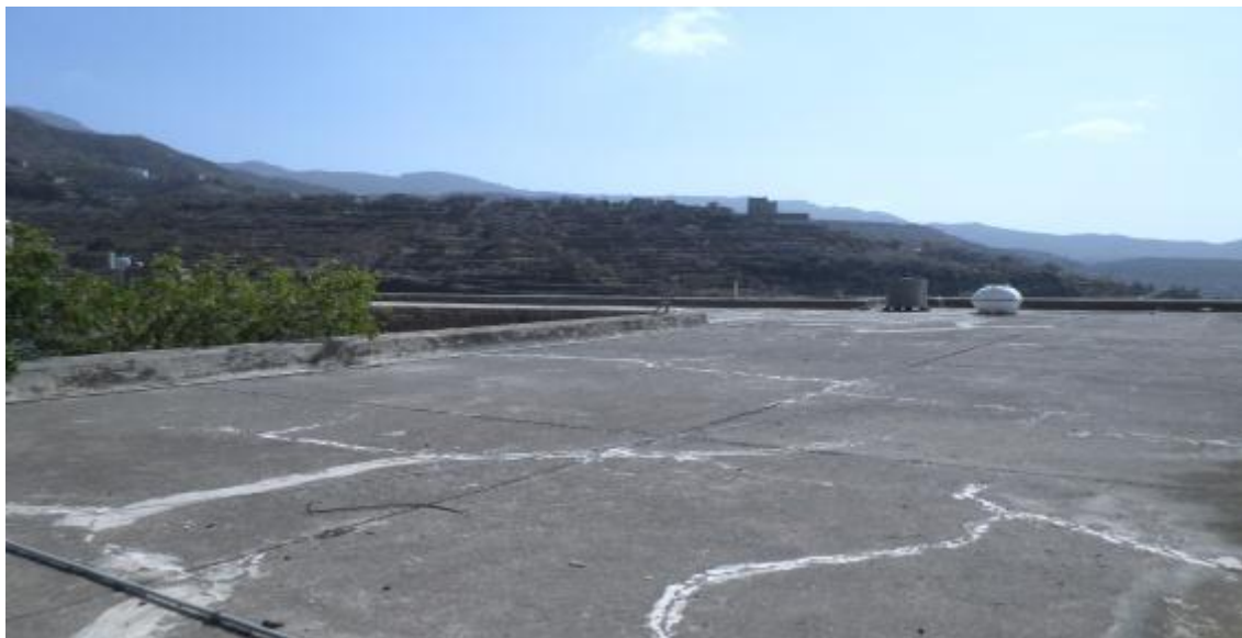
AL-MAWAST COUNTRYSIDE HOSPITAL Rooftop
