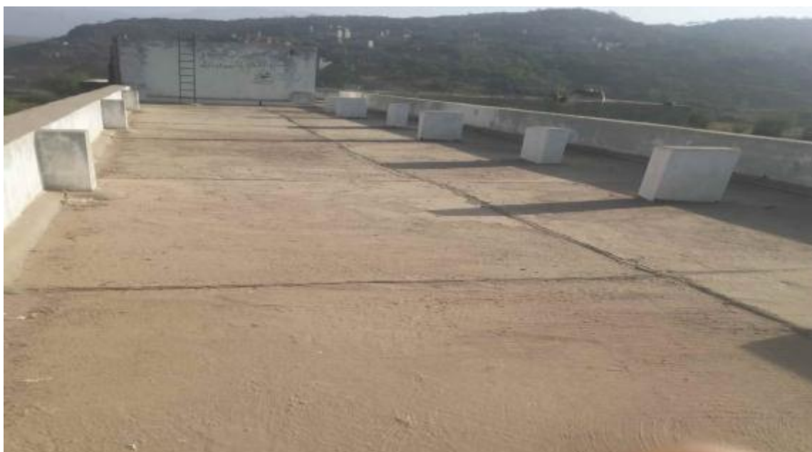
AL FAWZ SCHOOL ROOFTOP
