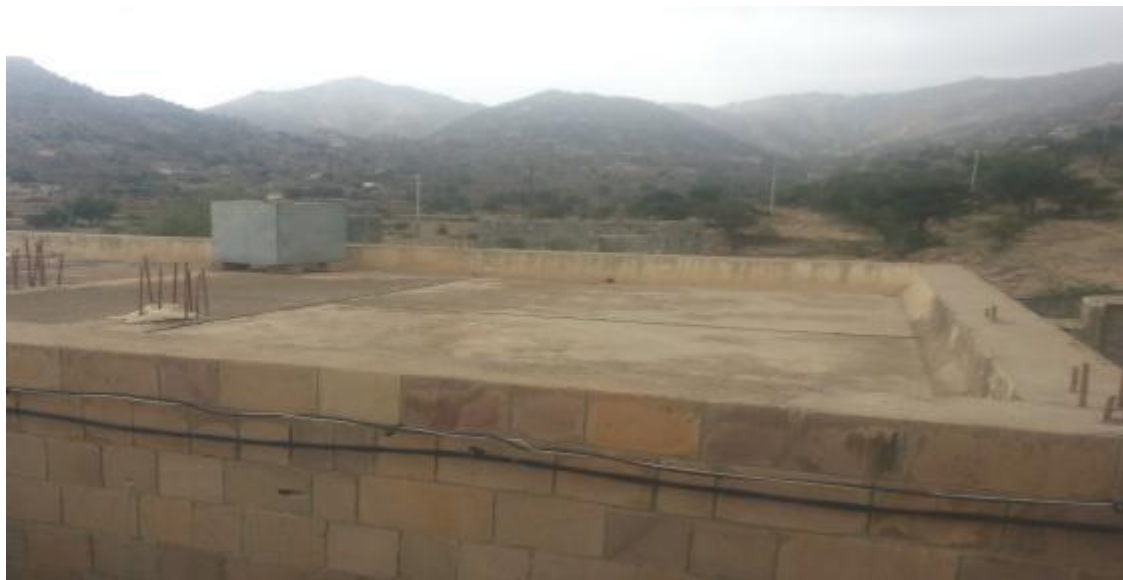
DA'AN HEALTH CENTER Rooftop
