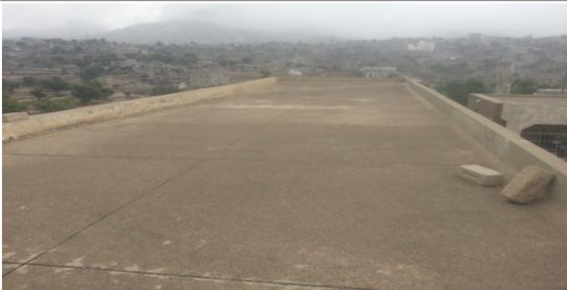
OMAR BIN ALKHATAB SCHOOL Rooftop
