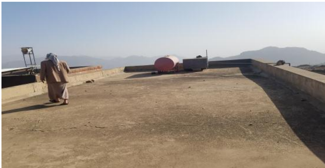
THEBA SCHOOL Rooftop
