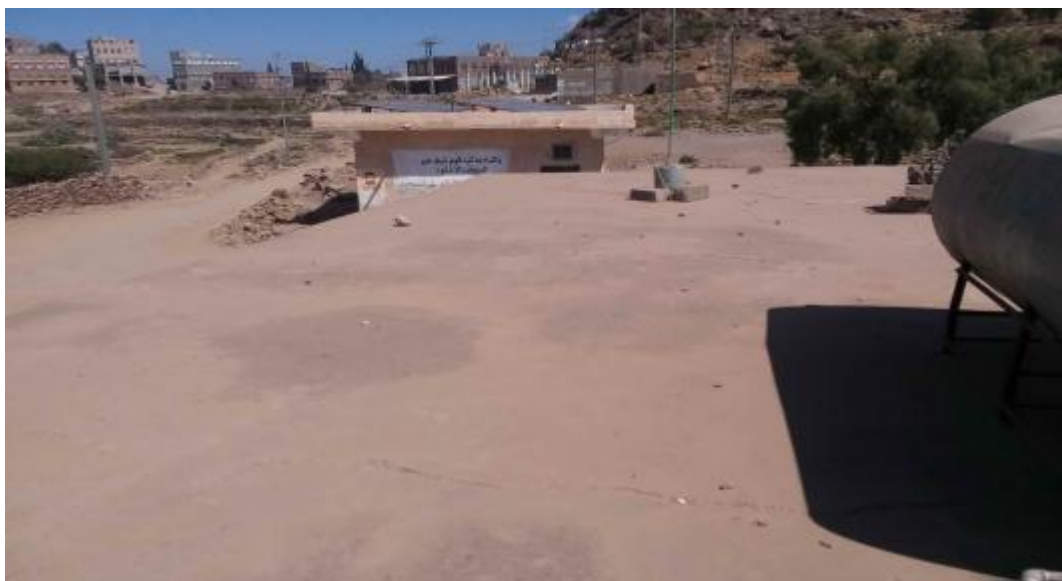
AL NAJAH SCHOOL ROOFTOP
