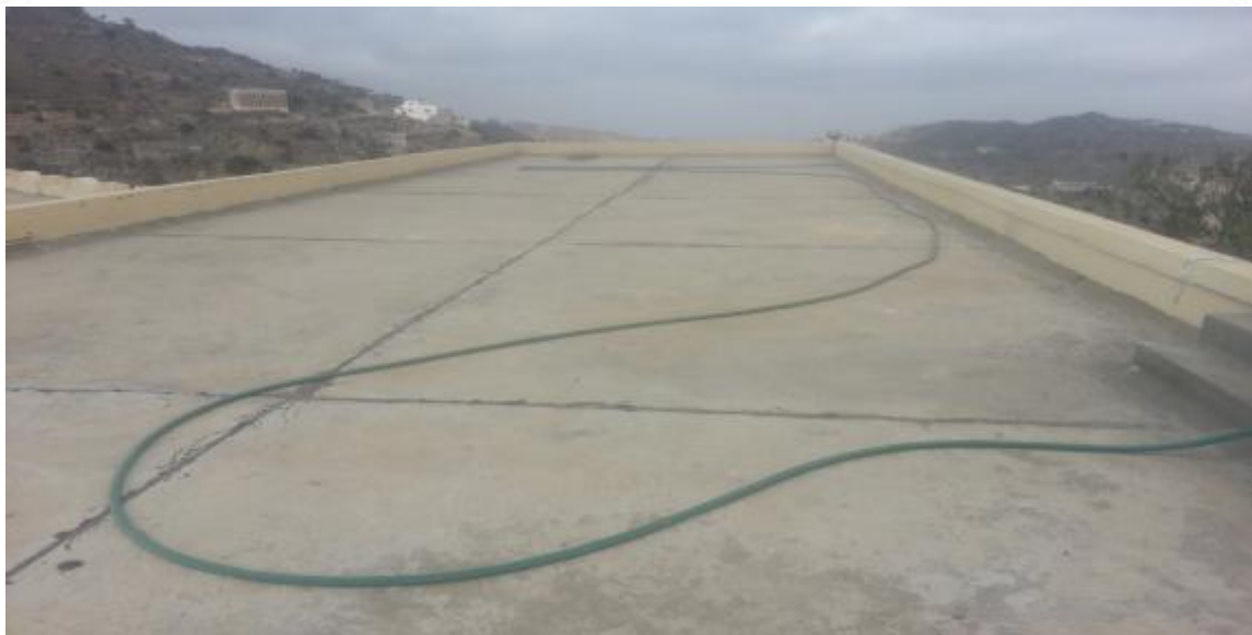
ALHATWA SCHOOL Rooftop
