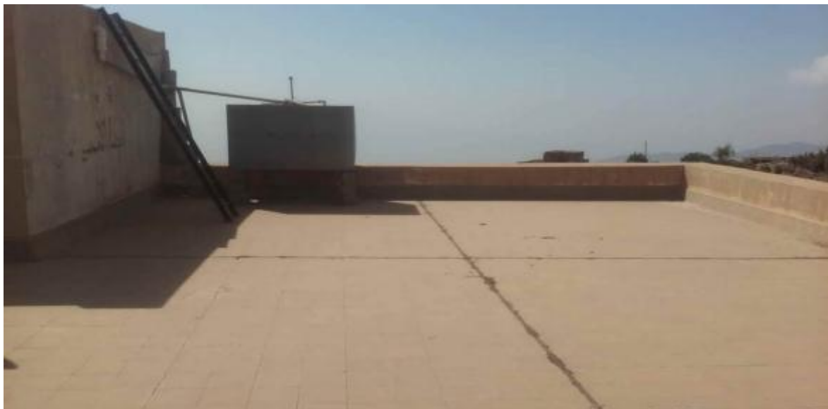
AL ADEL SCHOOL ROOFTOP
