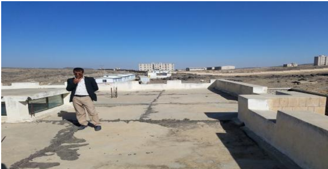
BANI QAOUS HEALTH CENTER Rooftop
