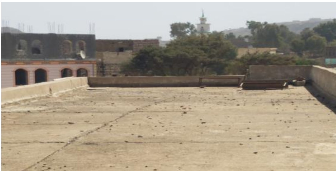
AL KHAREBAH HEALTH CENTER Rooftop
