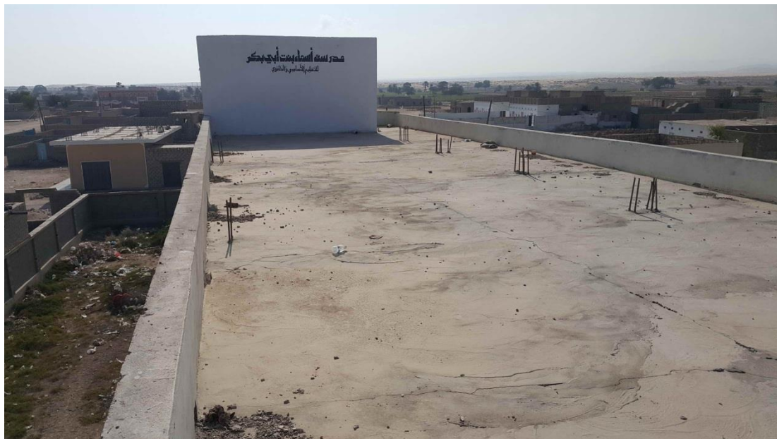
ASMA BINT ABI BAKE SCHOOL ROOFTOP
