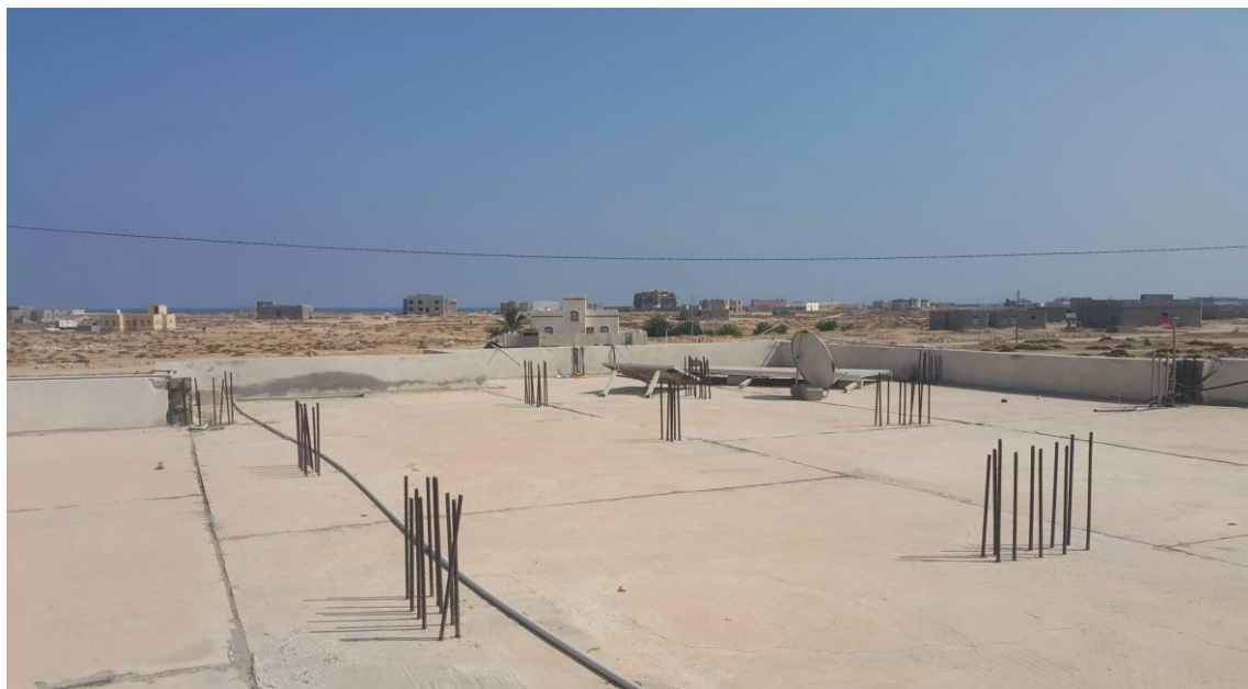
HASWAYN HEALTH CENTER ROOFTOP
