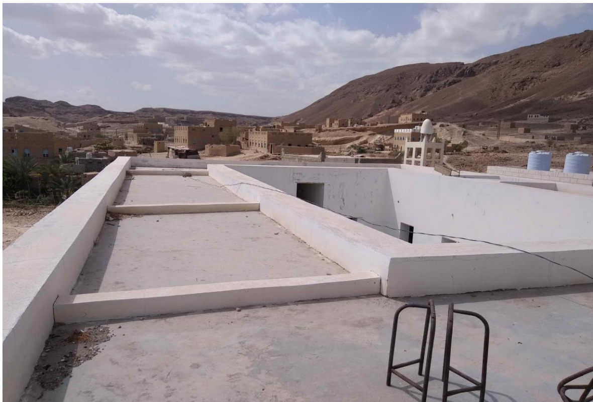
AMAR BIN YASER SCHOOL ROOFTOP
