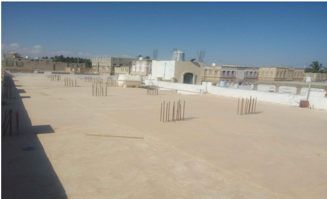
SHUHEER HEALTH CENTER ROOFTOP
