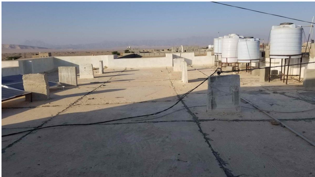
GAOL AL RAIDAH HEALTH CENTER ROOFTOP
