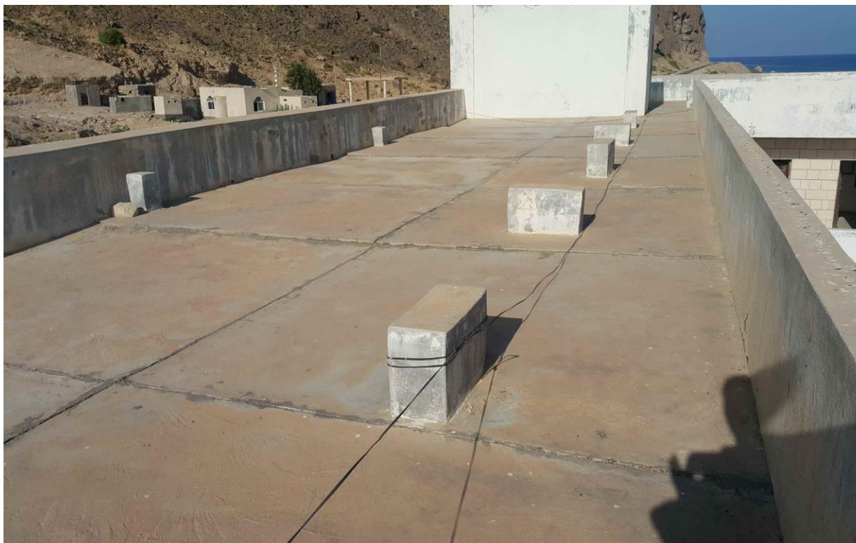
MADRAM SCHOOL ROOFTOP
