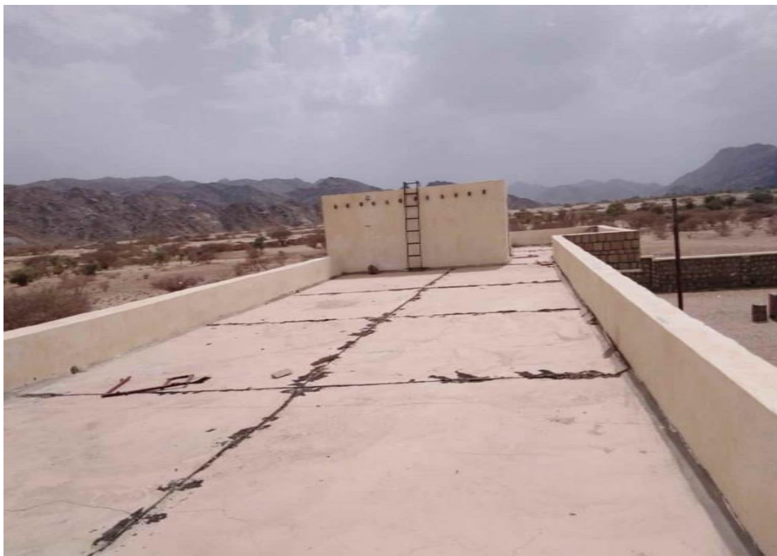
AMANGEL SCHOOL ROOFTOP
