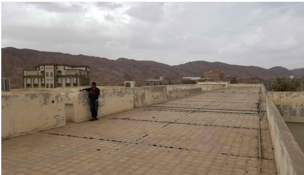
AL MUSENAH HOSPITAL ROOFTOP
