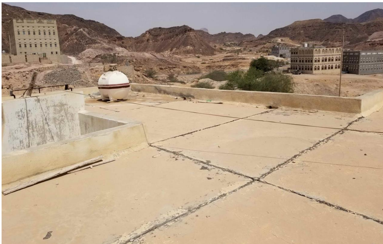
GHORAIER HEALTH CENTER ROOFTOP
