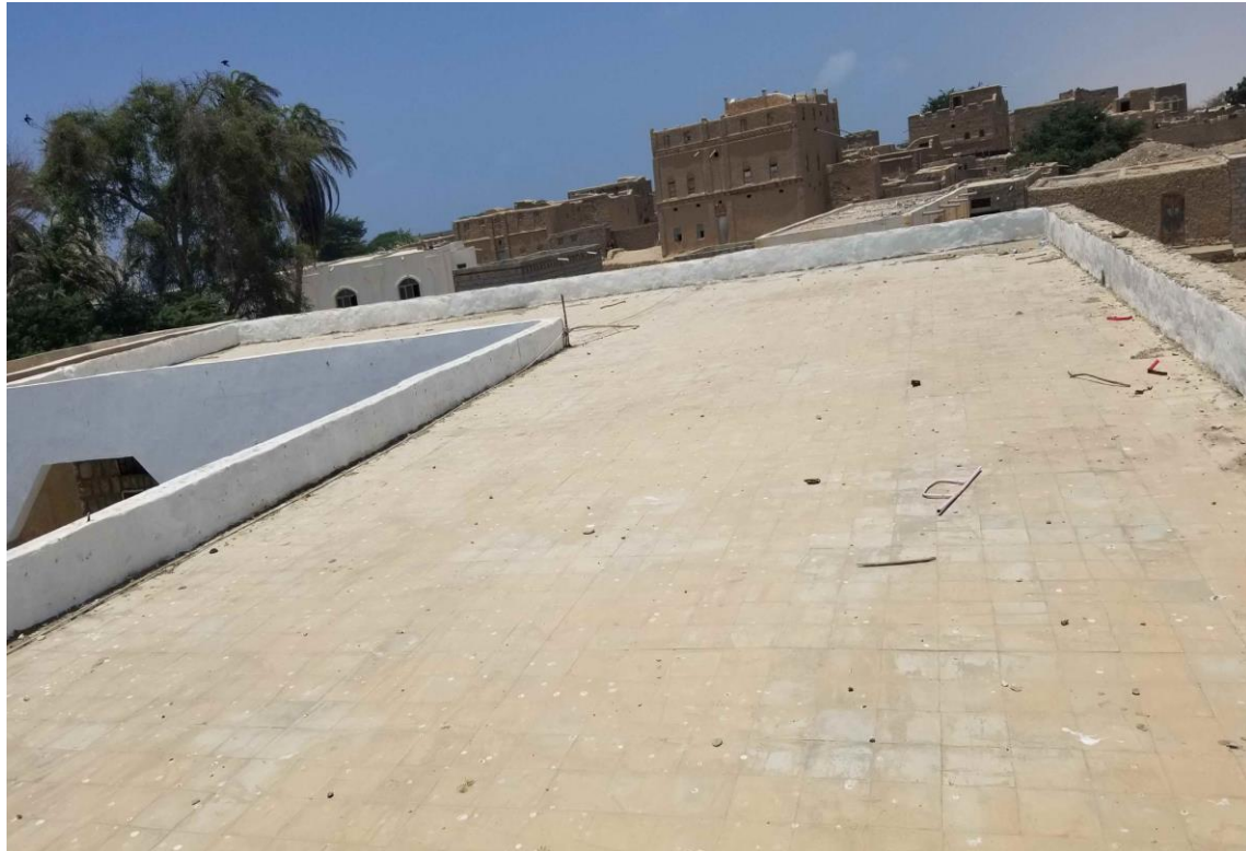
ARQAH SCHOOL ROOFTOP
