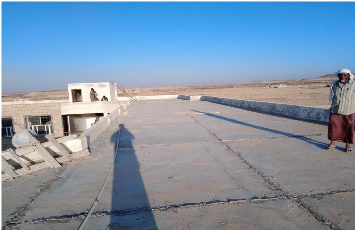
AL-TALIAH SCHOOL ROOFTOP
