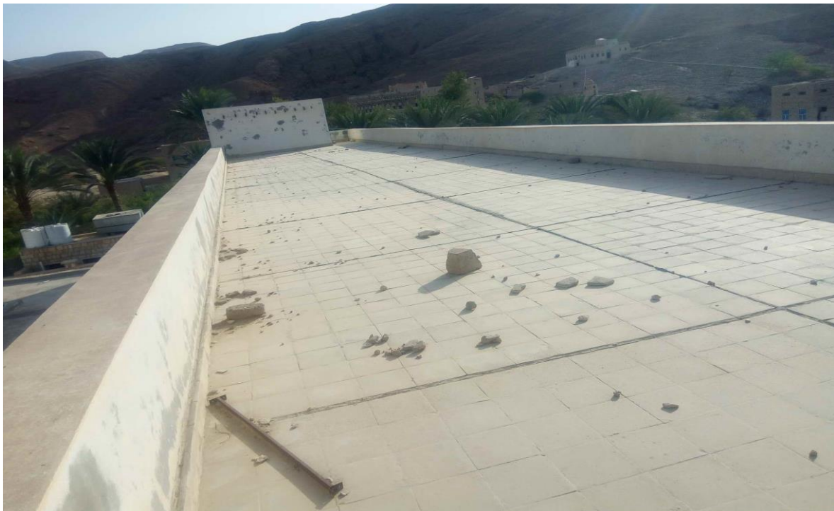
ALFAROK SCHOOL -ALSADARA ROOFTOP
