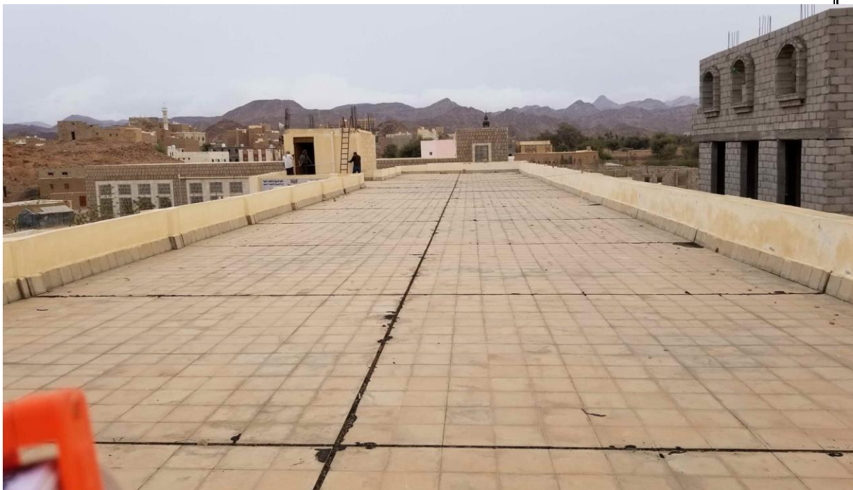
ALMUSIENAH SCHOOL ROOFTOP
