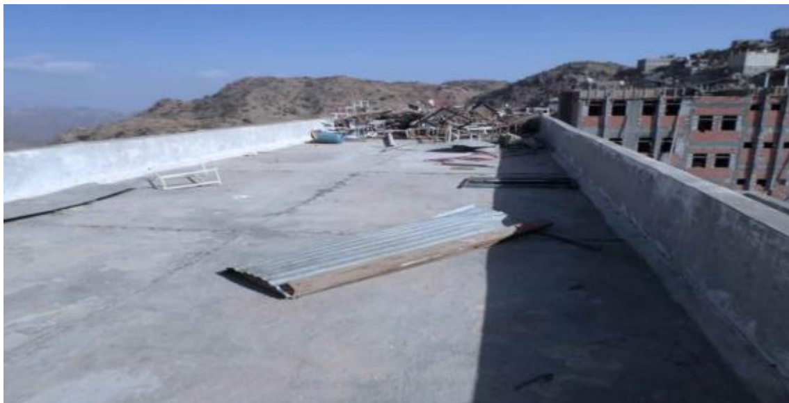
ZAINAB SCHOOL ROOFTOP
