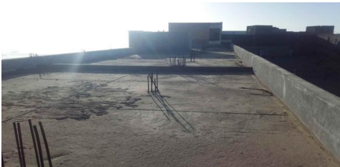
MARYAM SCHOOL ROOFTOP
