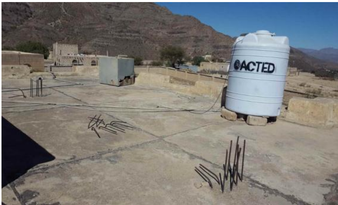
MUNERAH HEALTH CENTER ROOFTOP
