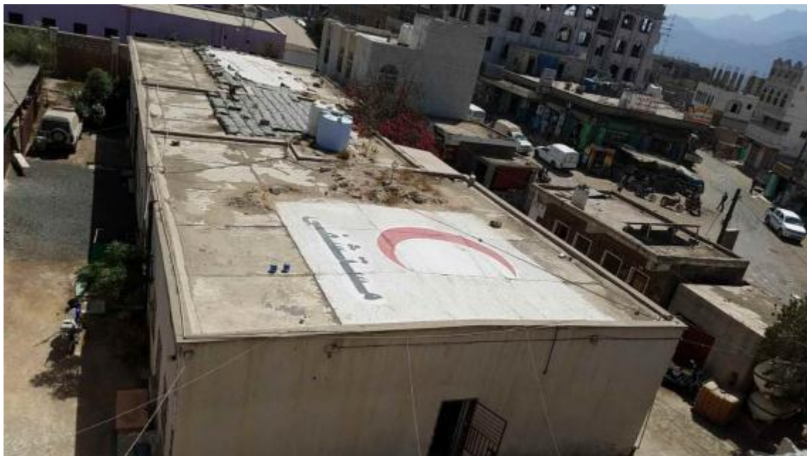
ALSALAM HOSPITAL Rooftop
