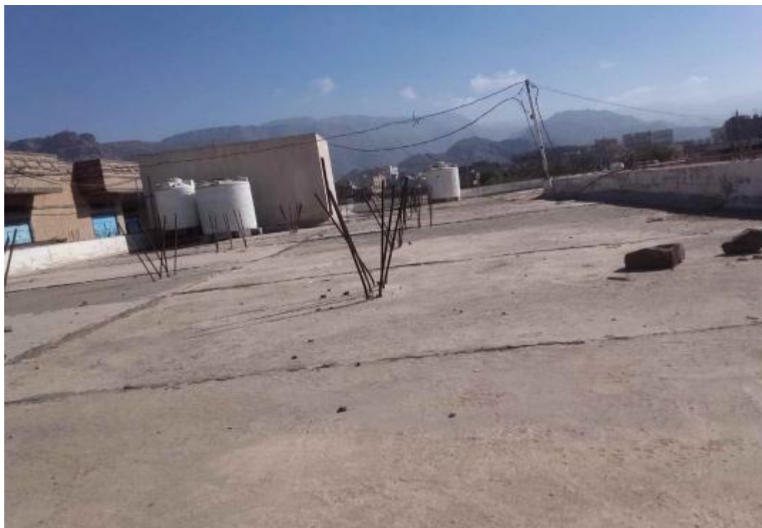
MATERNITY AND CHILDHOOD HEALTH CENTER IN QATABAH ROOFTOP
