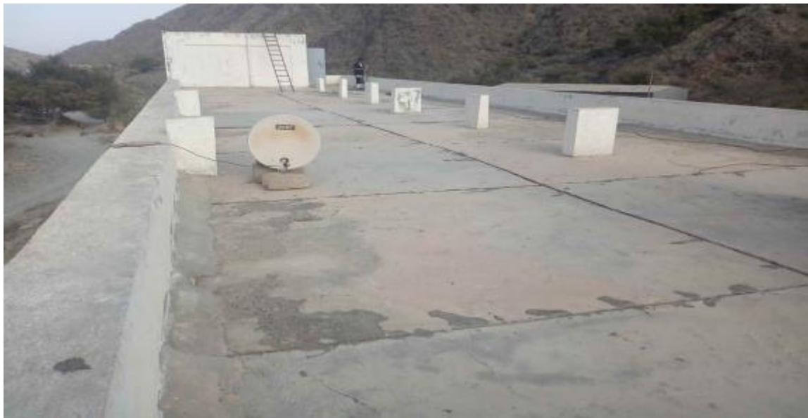
ALSA'EED SCHOOL Rooftop
