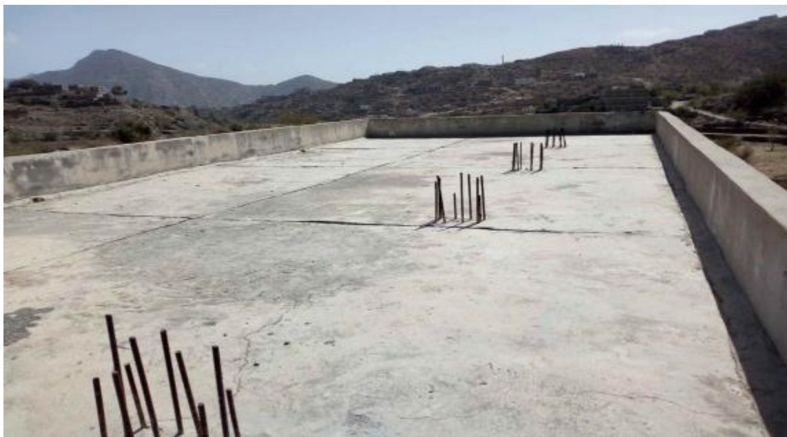
SALEM SALEH SCHOOL ROOFTOP
